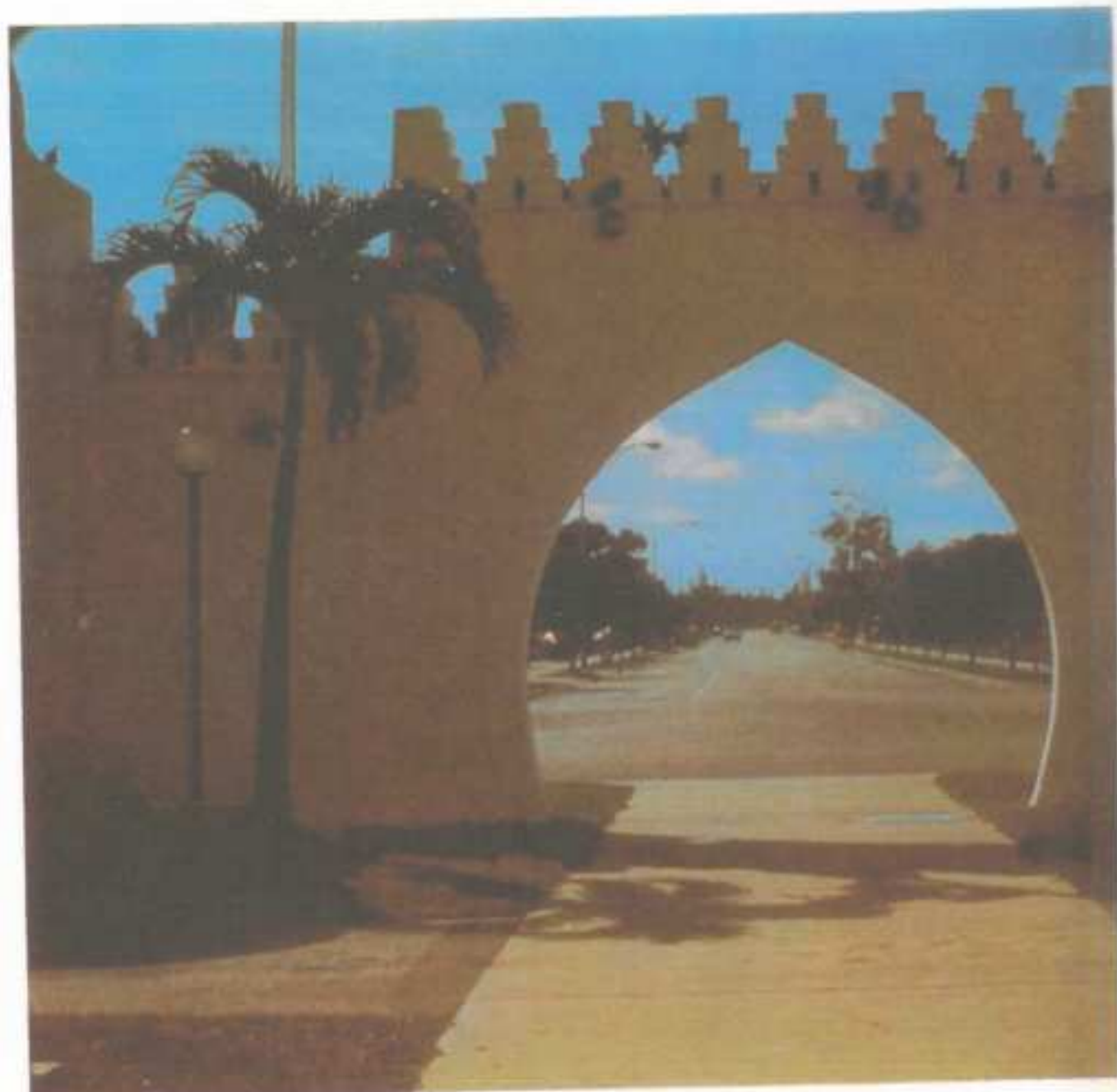
City Hall entrance gate, Opa-locka
