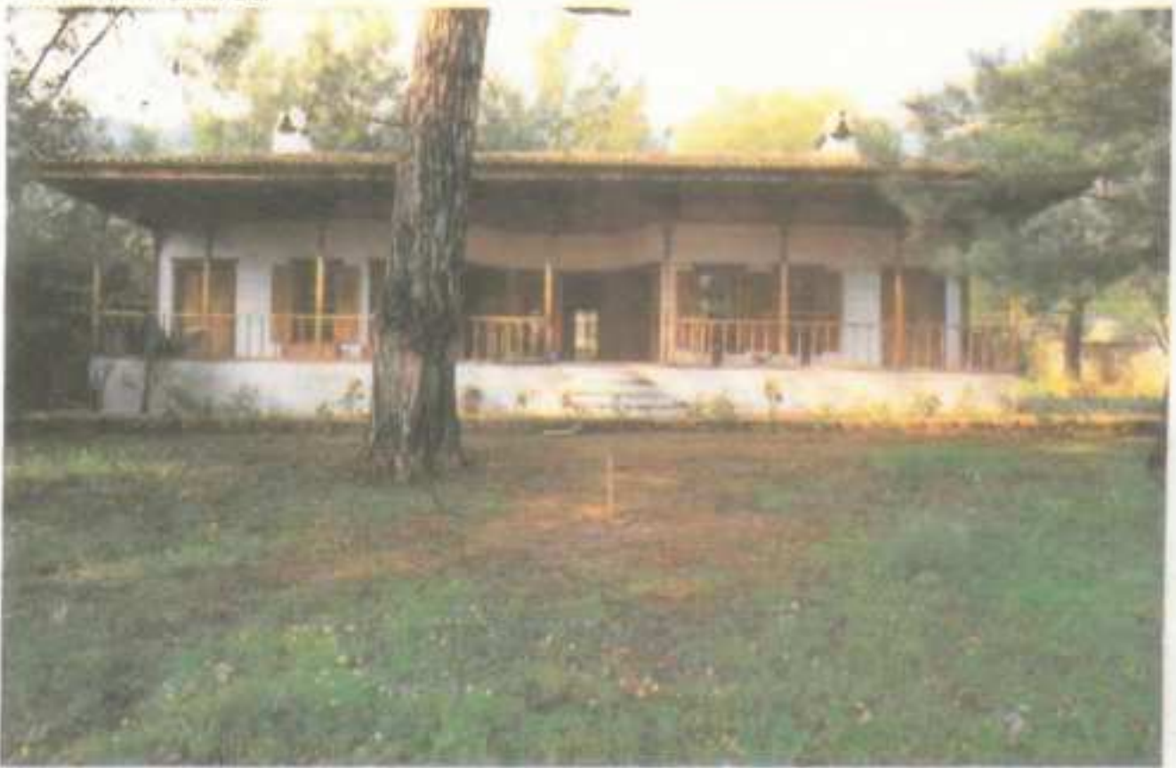
Nail Cebirhan Residence, Akya Village
