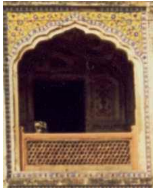
The Detail of balcony, on the right bay of the main façade.
