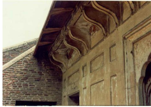
Brackets on the 1 st floor.
