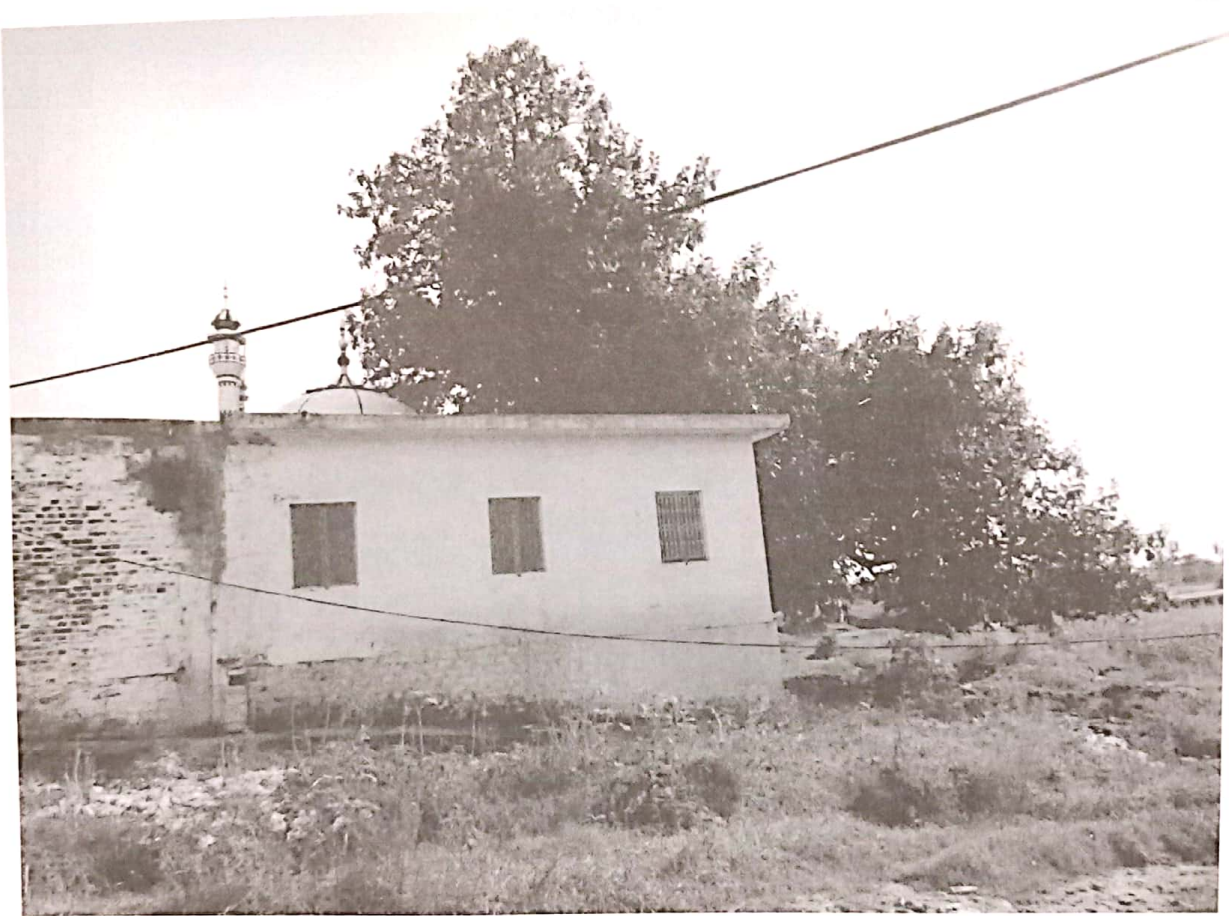
Fig. 9 - Akbari Masjid after the renovation (1994).
