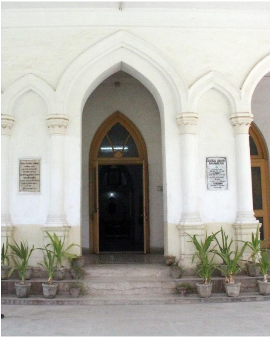
Figure 25. Entrance door of the Central Library. Source: Picture by Author.
