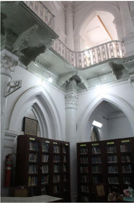
Figure 29. Double arches in the internal hall. Source: Picture by Author.
