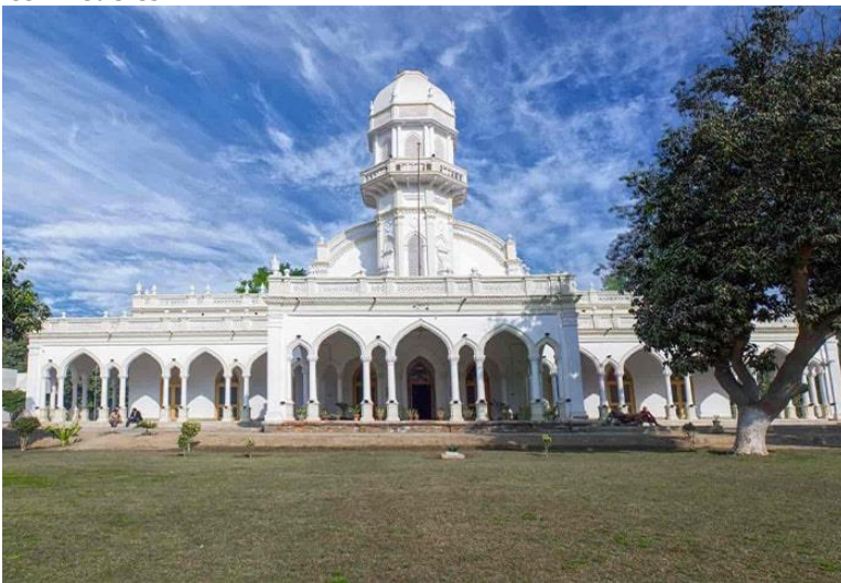
Figure 1. Front Facade of the Sadiq Library 1924. Source: Picture by Author.
