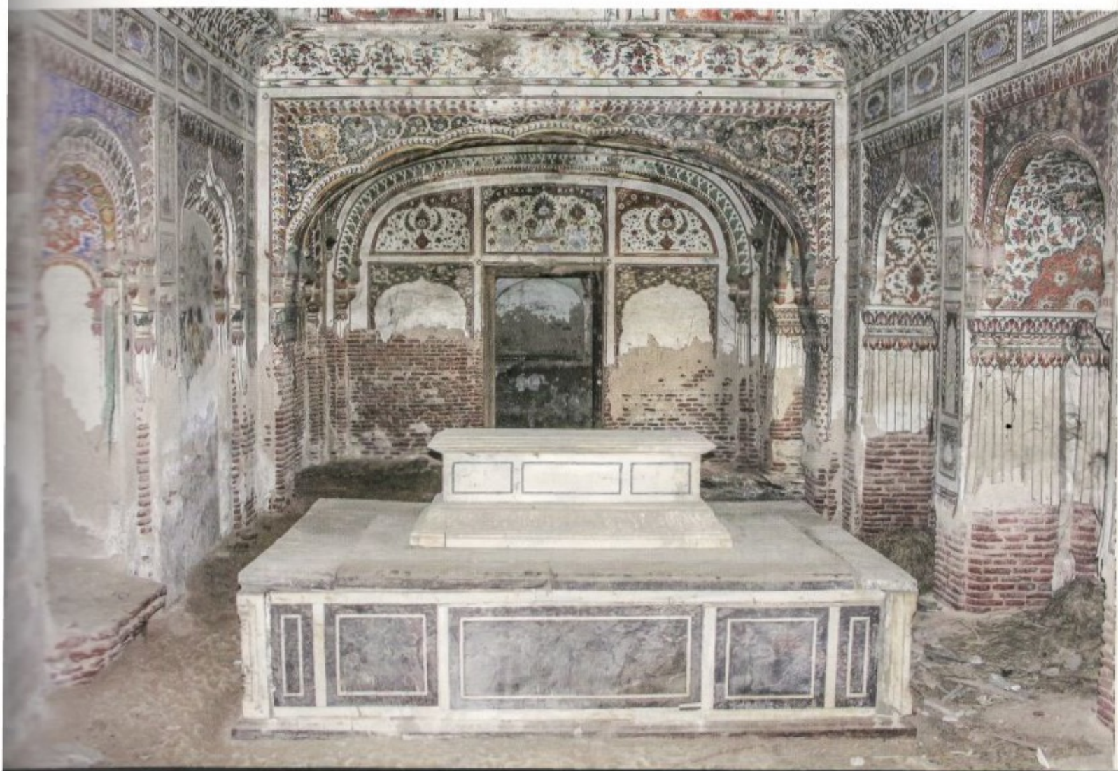
Fig. 21.7 The central rectangular room separated from the smaller side ones by archways on piers
