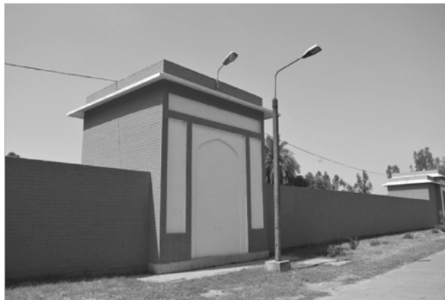
Figure 9. Western wall around the tomb Source: Photograph May 6,2023
