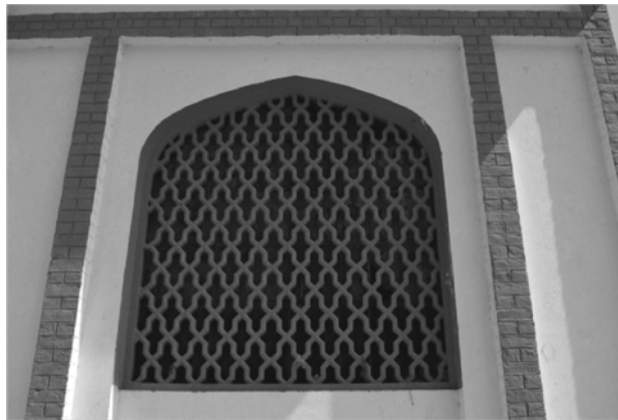
Figure 7. Details of terracotta lattice or jali work on the façade of the eastern walls Source: Photograph May 6, 2023
