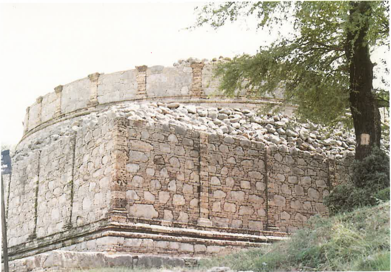
Closer view of the Stupa
