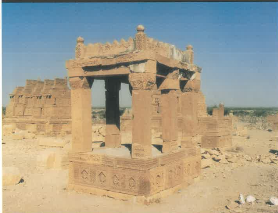
General View of a square canopy from Chaukhandi
