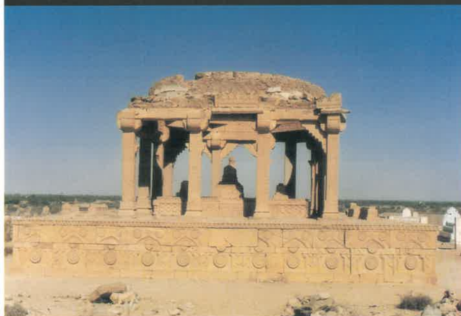
General View of a pillared canopy from Chaukhandi Graveyard.
