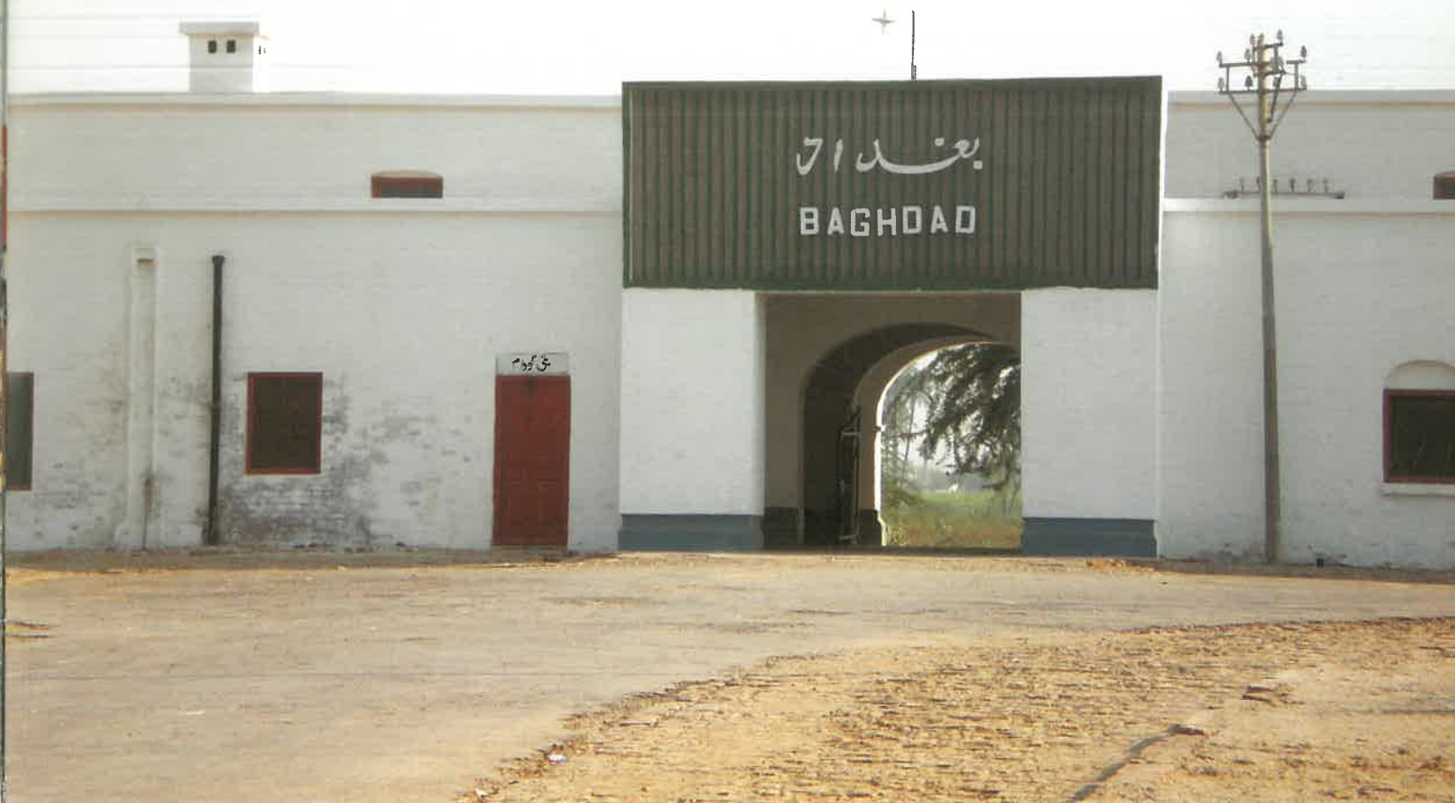
Baghdad Railway Station, Bahawalpur
