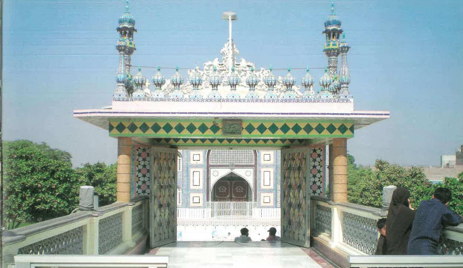
Entrance on Main Gate side
