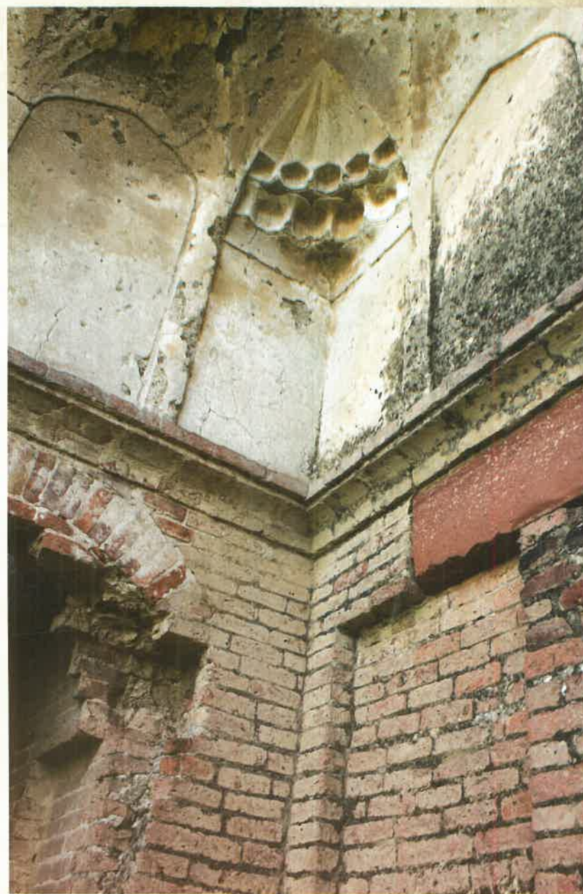
Squinch arch comprising honeycomb.
