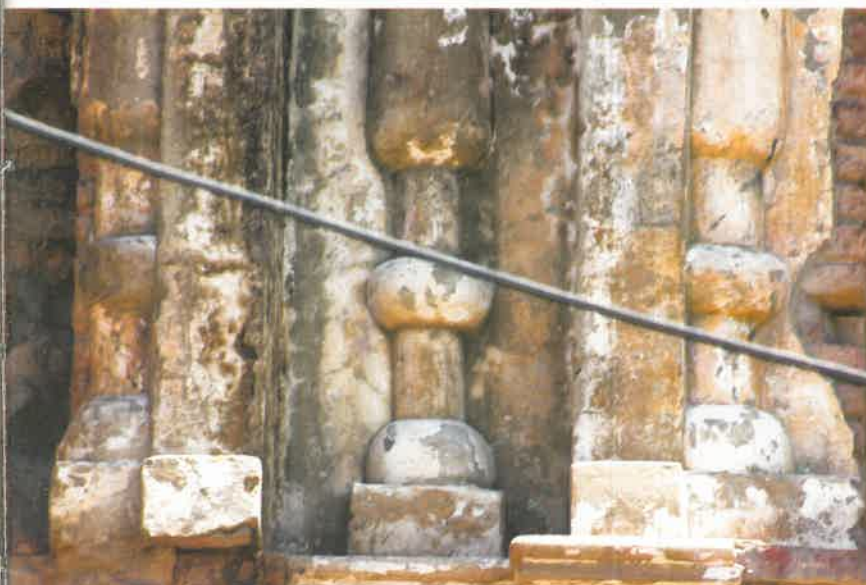
Miniature attached columns, water disposal units and corner garrets of the Kotha Sahib.
