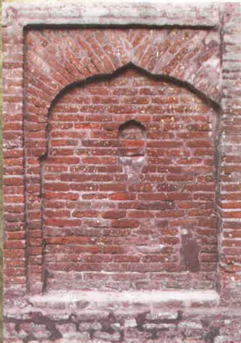
Depressed panel with a niche.
