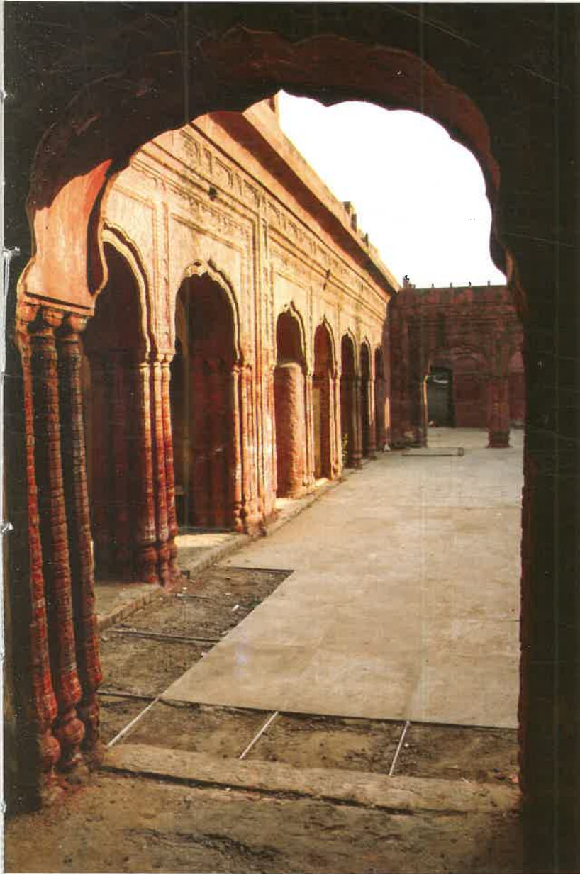
One of the cusped arches.
