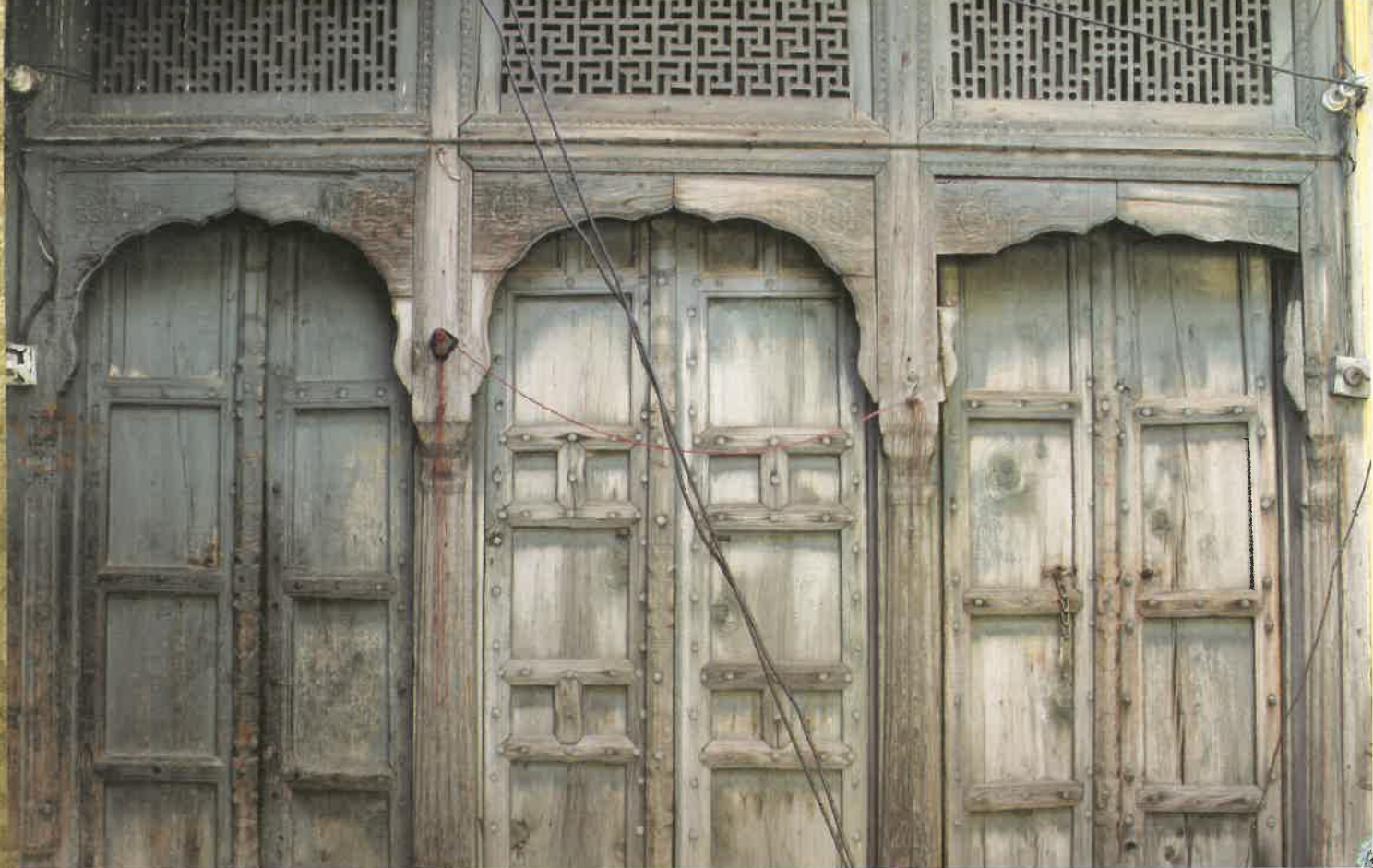
Internal wooden door Multifoil arches and trellis work.
