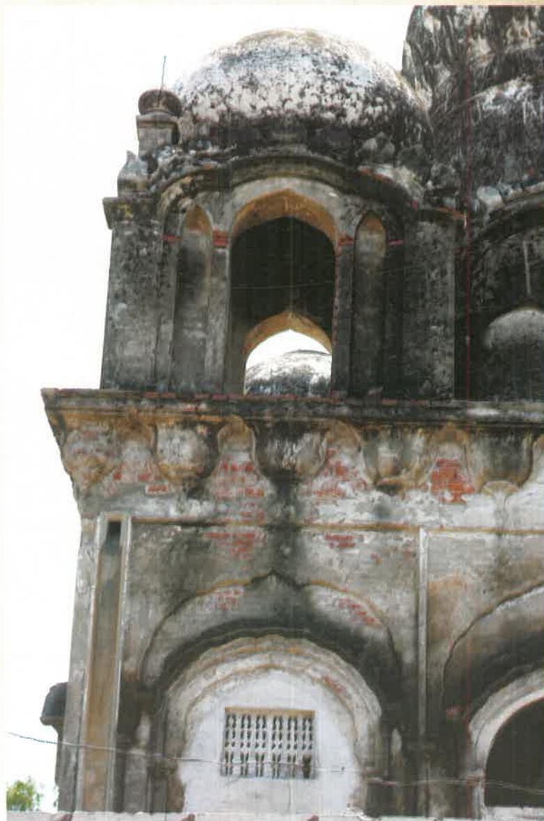
Miniature attached columns, water disposal units and corner garrets of the Kotha Sahib.
