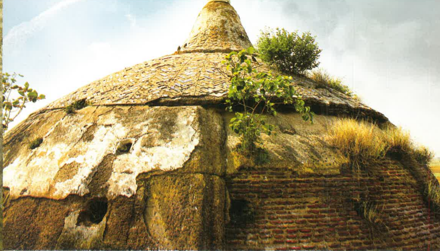
Surviving tilework on the apex of the dome and turrets.
