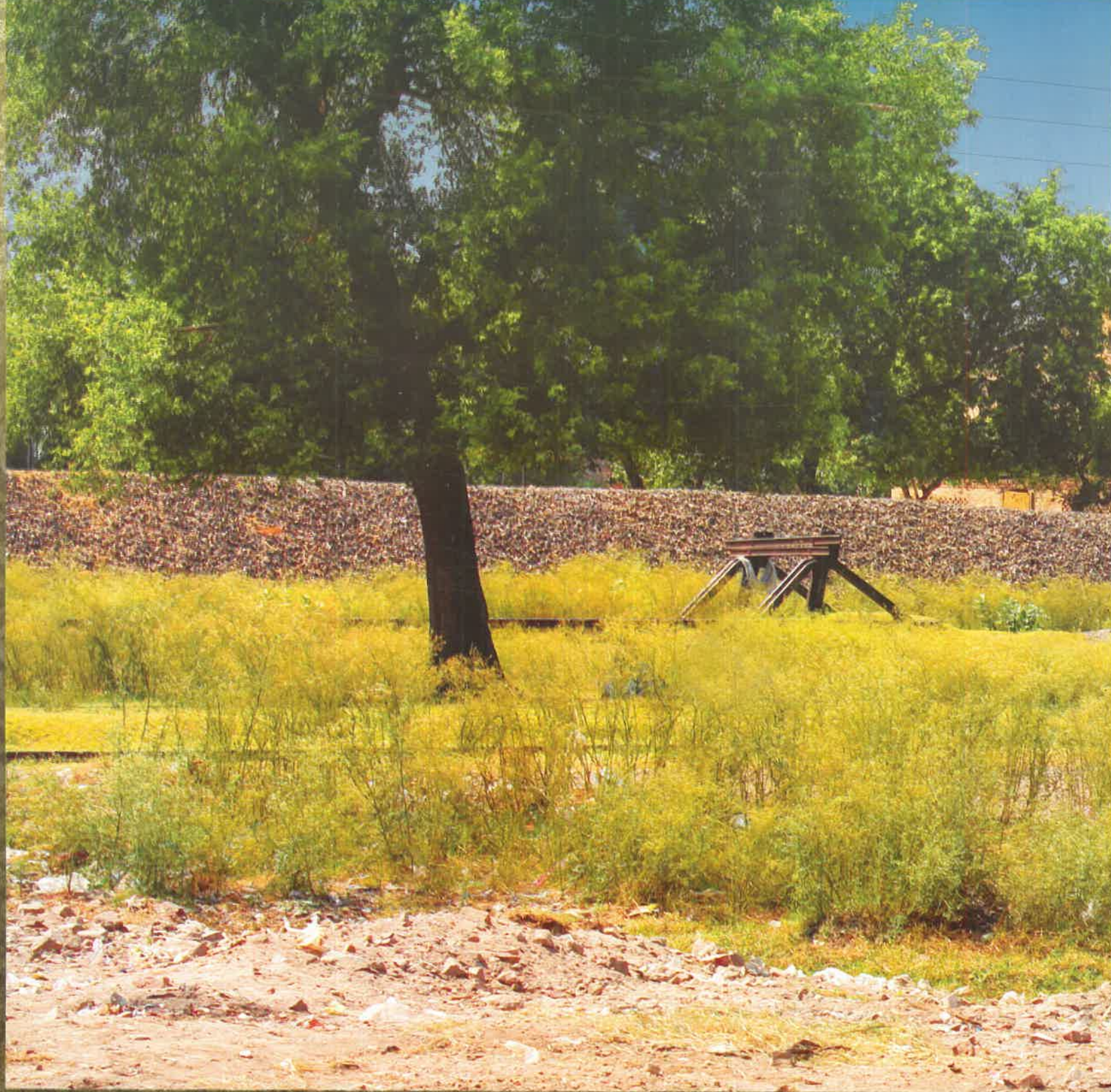
Wazirabad: Abandoned section of the Railway Station
