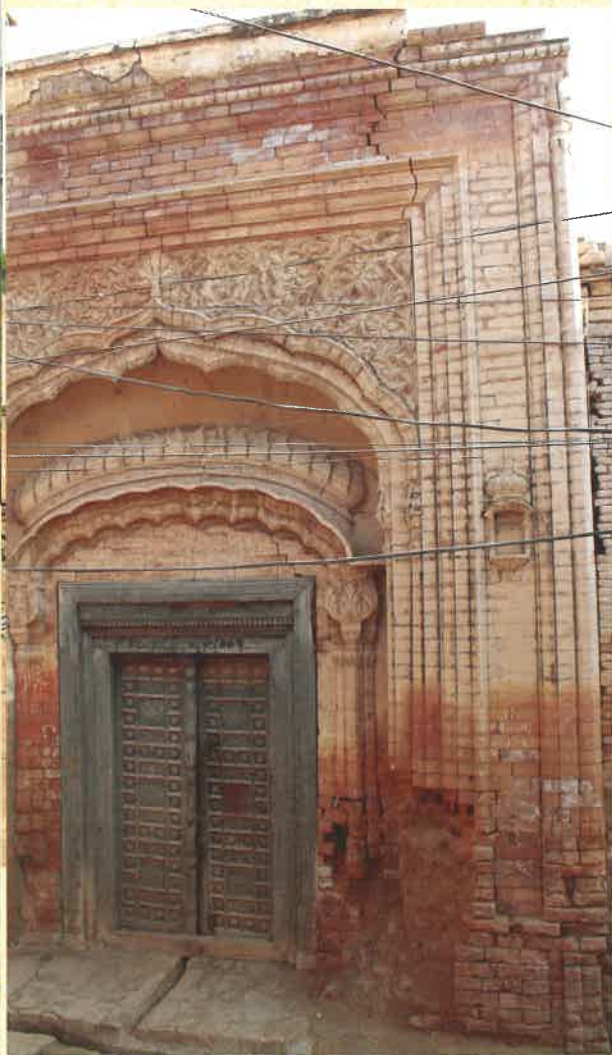
Farooka – exterior view of an old house with intricate patterns cut in hand molded & carved bricks.
