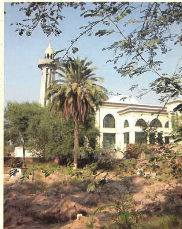
La'al Sharif near Mangowal. A new mosque built near the historical tomb of Shah Yousuf.
