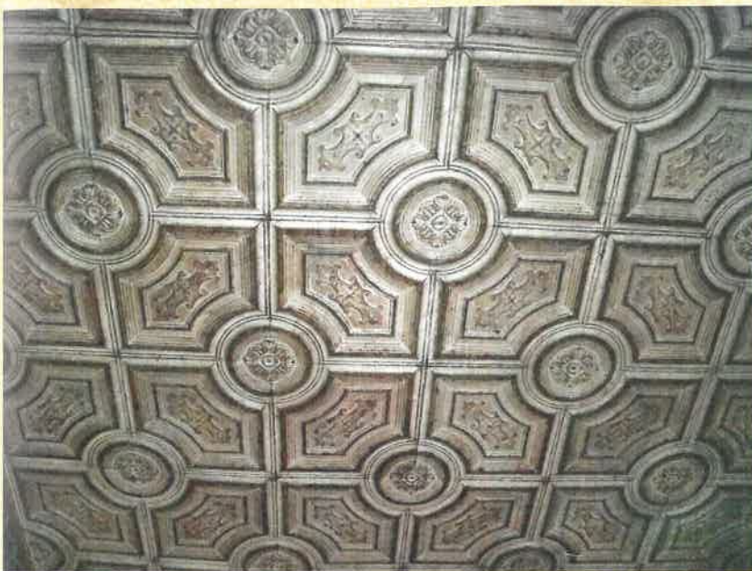
Miani –False wooden ceiling in one of the rooms of Krishna Niwas.
