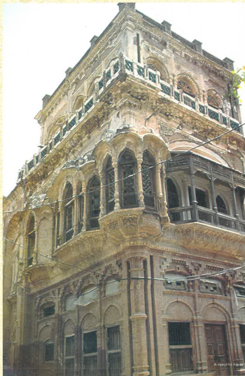
Bhera – A beautiful multi storey traditional house in Mohalla Saniah Wala. Photo 1988
