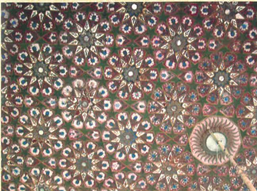
Bhera –False wooden painted ceiling in a mosque.
