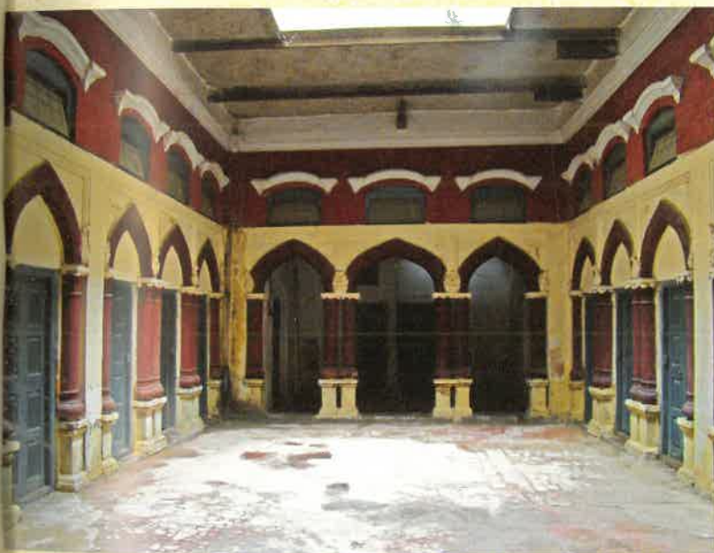
Miani – Krishan Niwas (1928) interior of the building.
