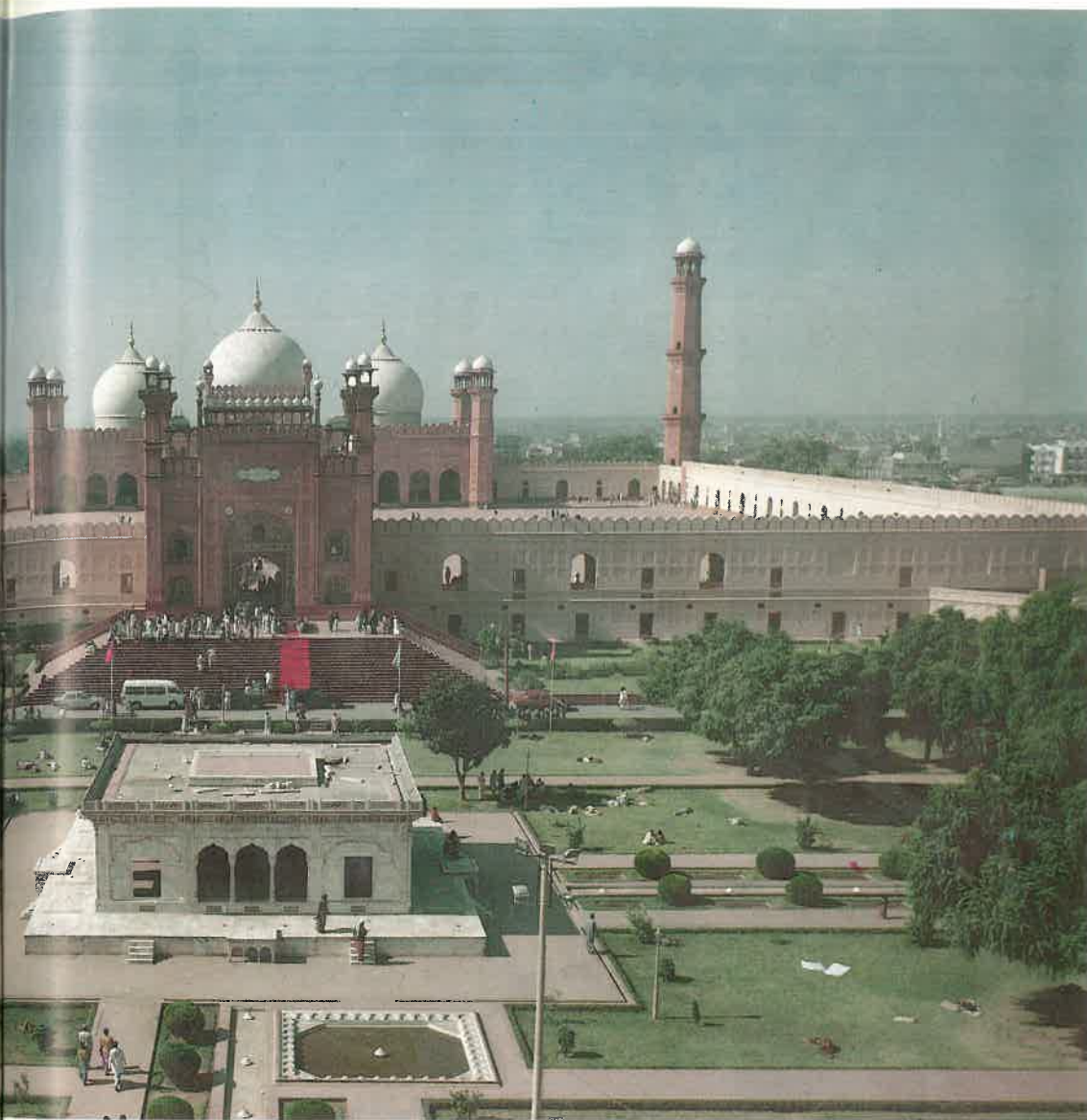
Pl. 57 The Badshahi Mosque, Lahore: General view from the Hazuri Bagh.
