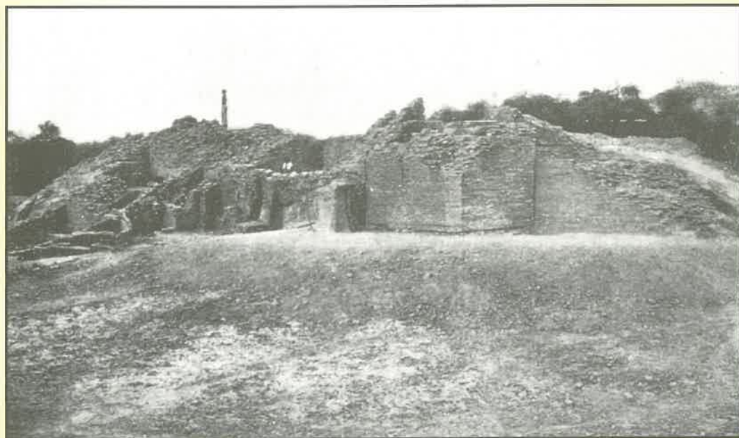
Moenjodaro: Group of towers at southeast corner of citadel
