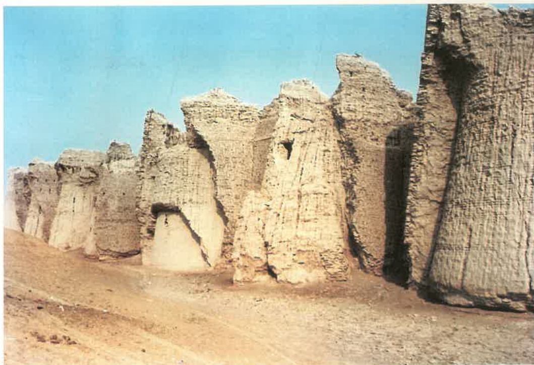
Maujgarh Fort : Wall And Bastions
