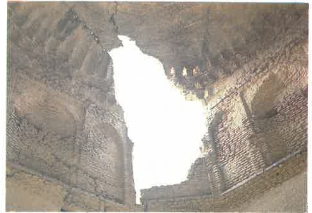
Interior of the dome showing cut brick corbelling.
