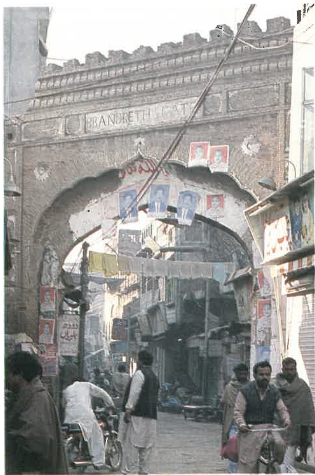
Brandreth or Sialkoti Gate; the only gate that survives out of eleven.
