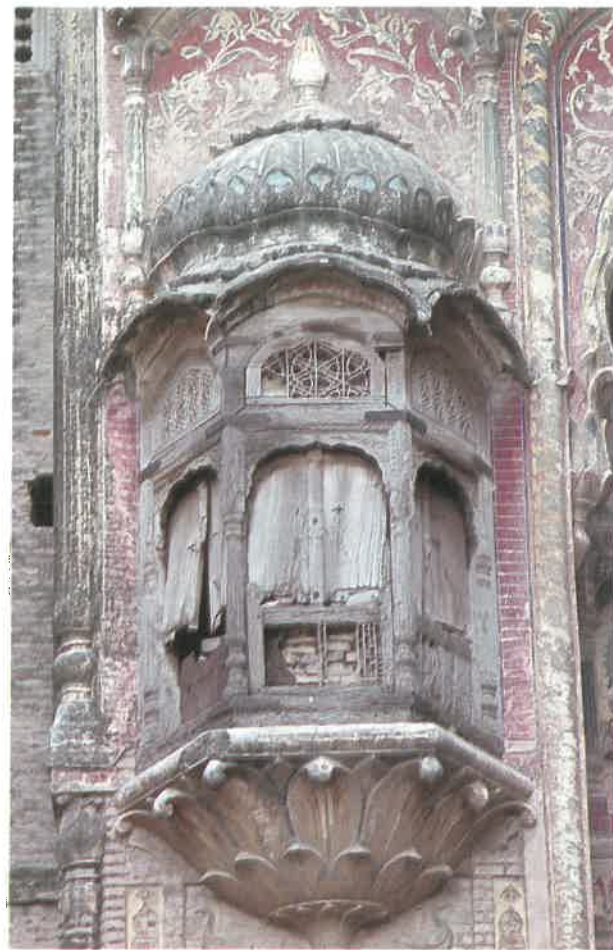
Detail of bay window.
