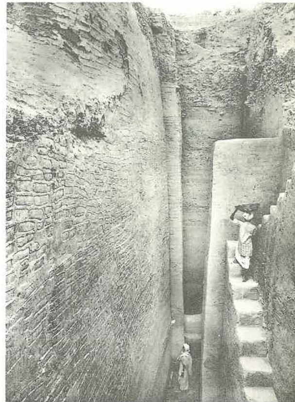
Section of the mud-brick wall on western side of the citadel.
