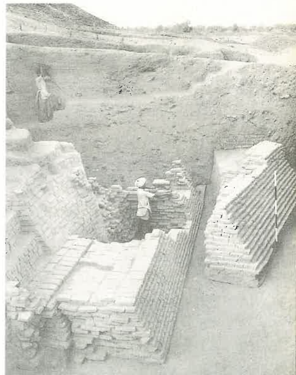
Baked brick revetment of mud-brick defensive wall of citadel.
