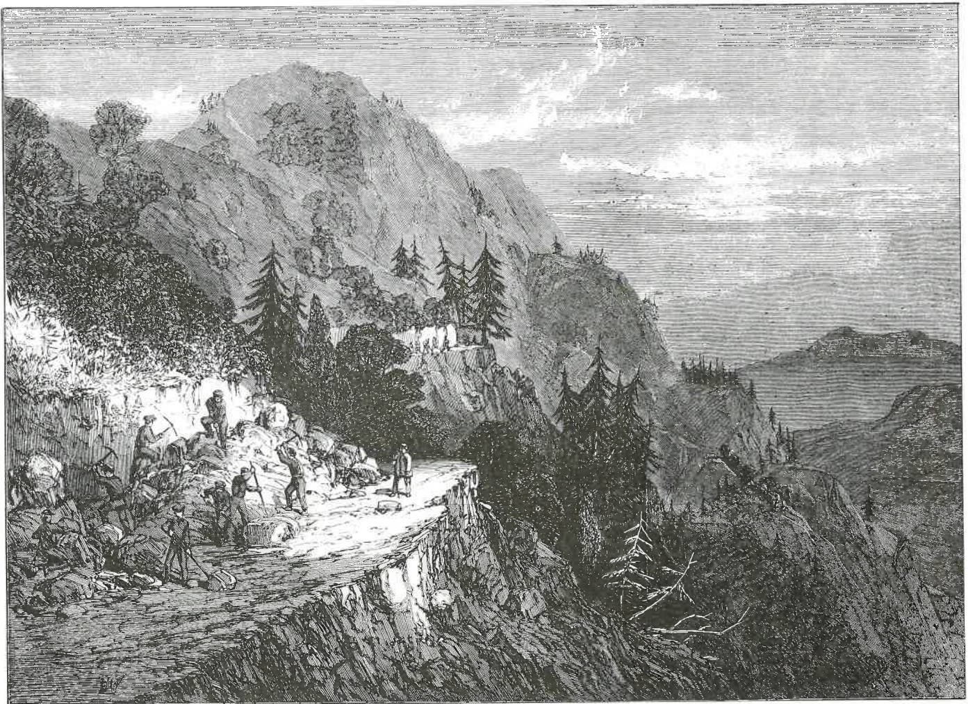
189 Roadmaking in the Murree hills, 1863.
