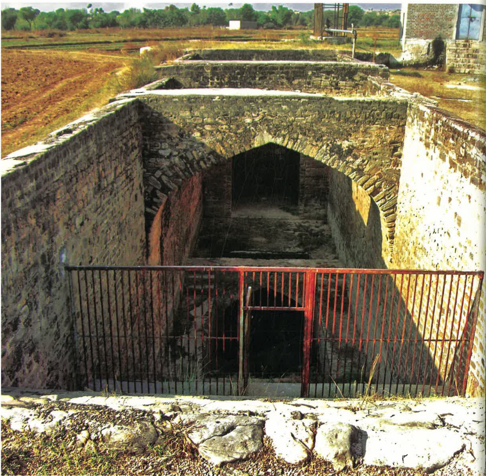
The steps leading down to the water level in the Khukha baoli. The concrete structure on the upper right corner is the pump room that supplies water to several surrounding villages.
