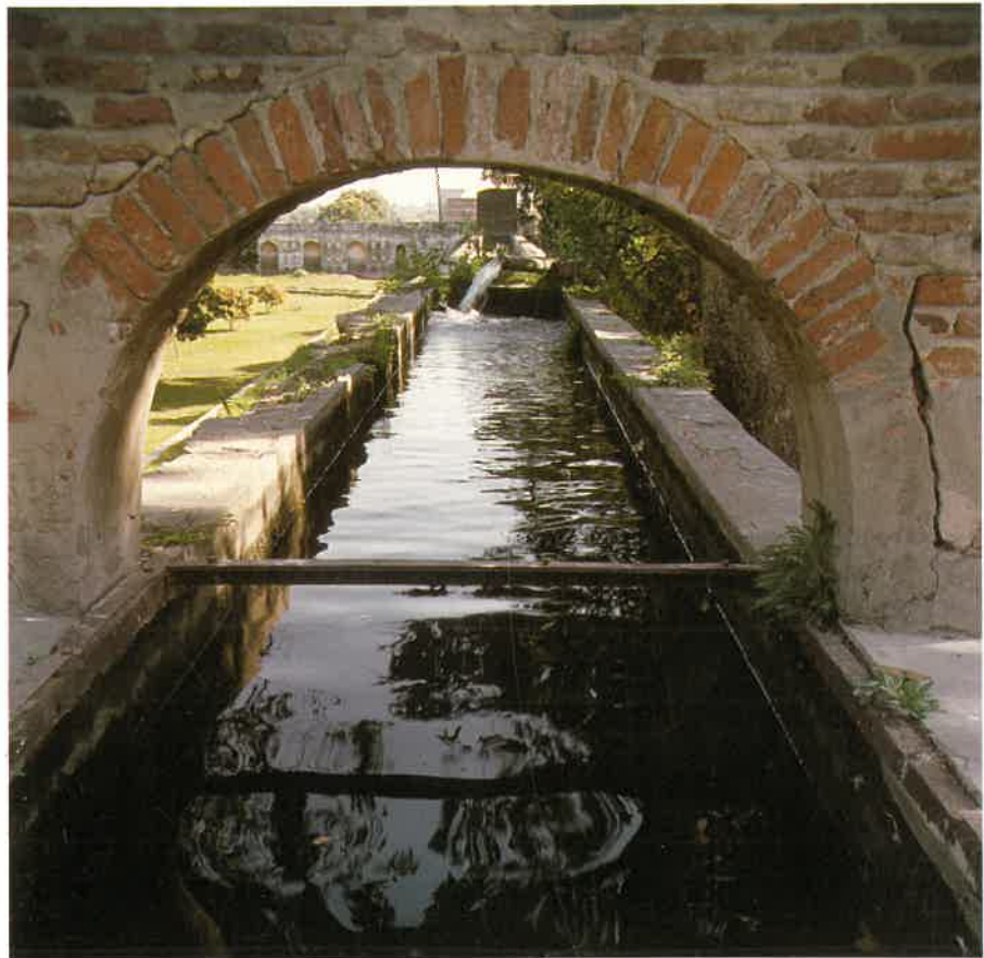
Jahangir's Tomb: Water-channel running over the top of the wall.
