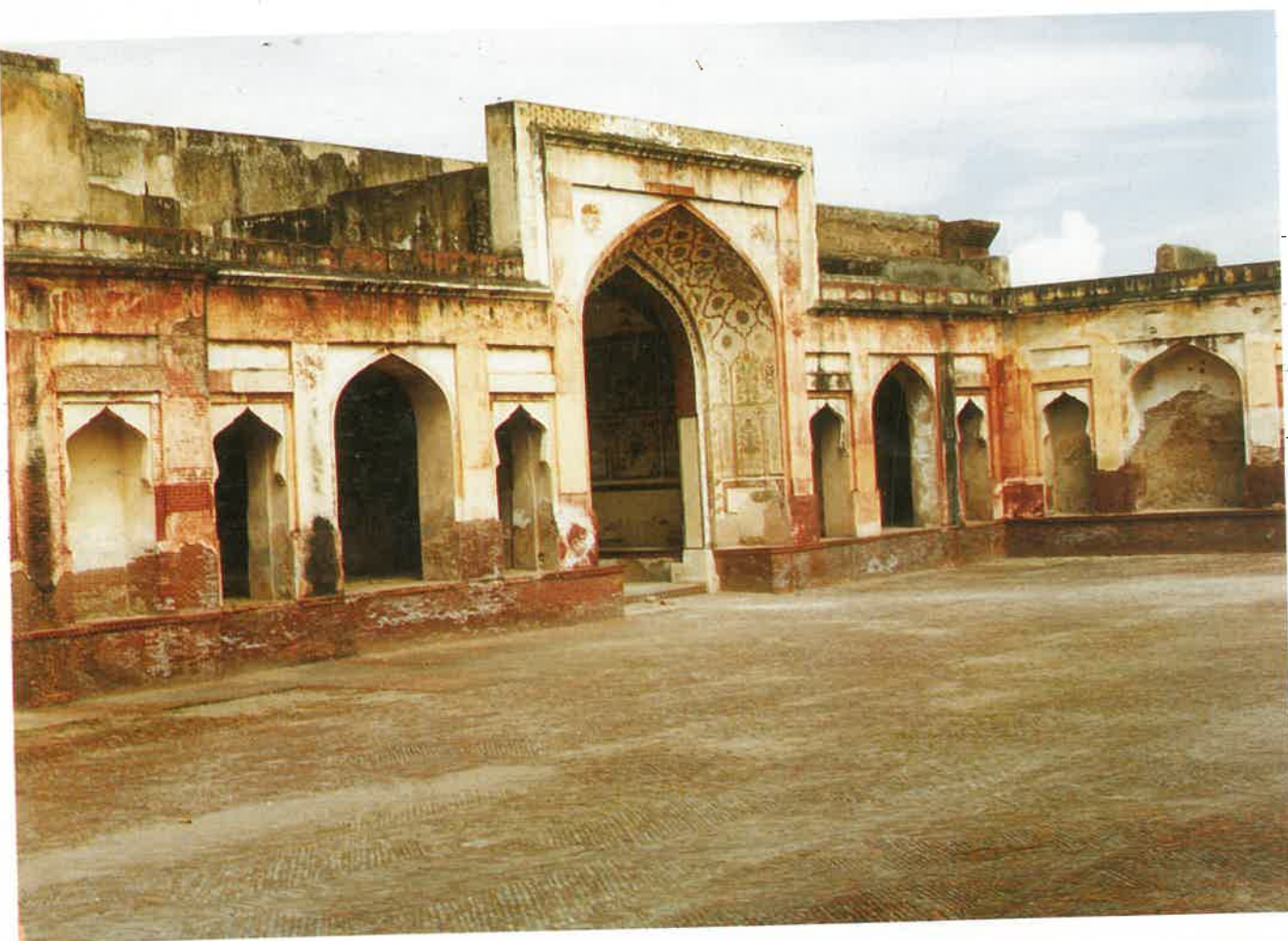
Entrance to the Shish Mahal Fore Court.
