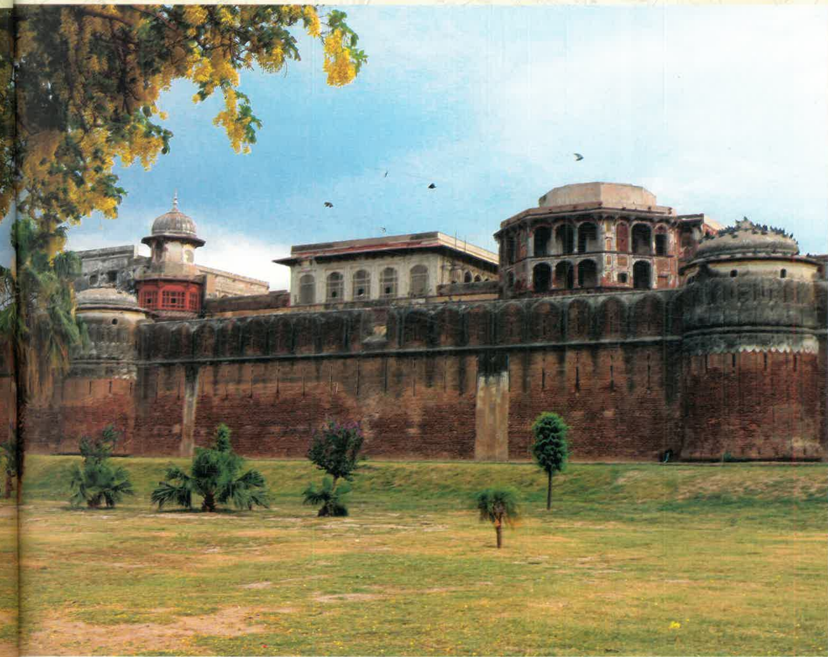
Exterior wall of the Lahore Fort.
