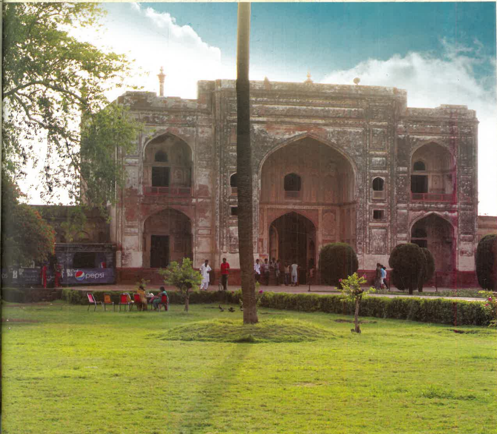
Eastern façade of main gate of Jahangir's Tomb
