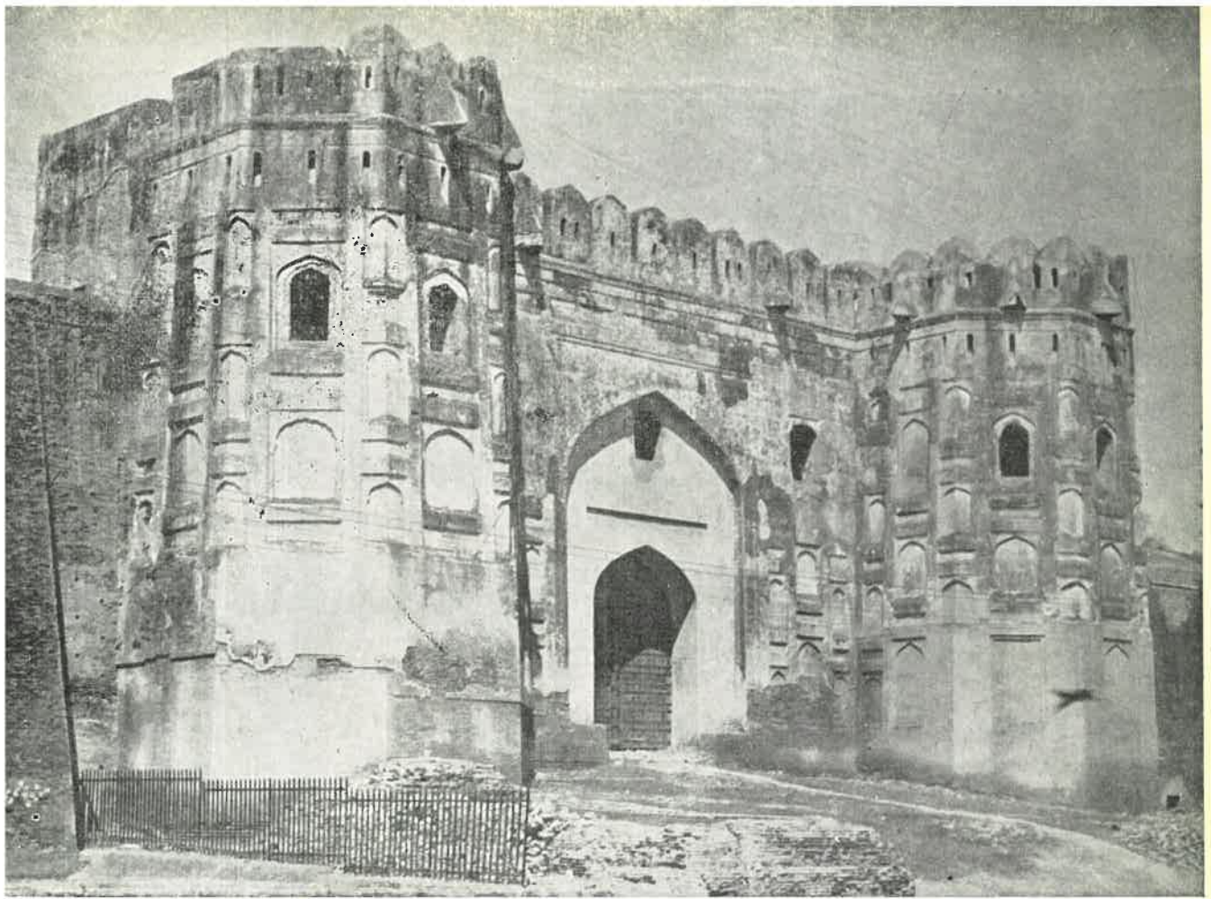
Masjidi or Masti Gate, Lahore Fort, built by Akbar in 1566 A.D.
