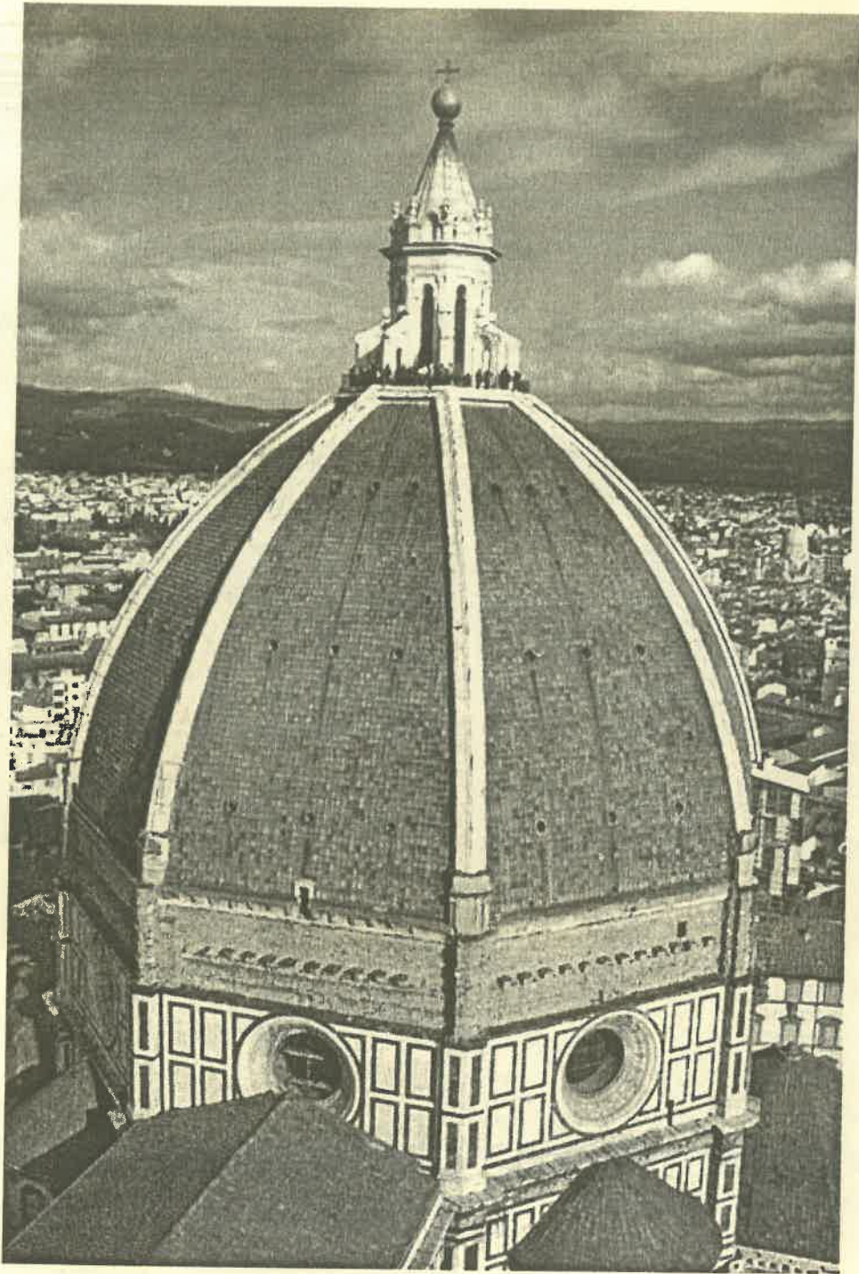
Filippo Brunelleschi, Dome for the Duomo of Florence , 1436, Florence, Italy
