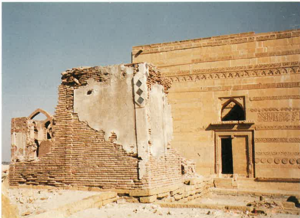
White plastered brick tomb south of tomb of Jam Nizamuddin. Part of old mosque at left also visible.
