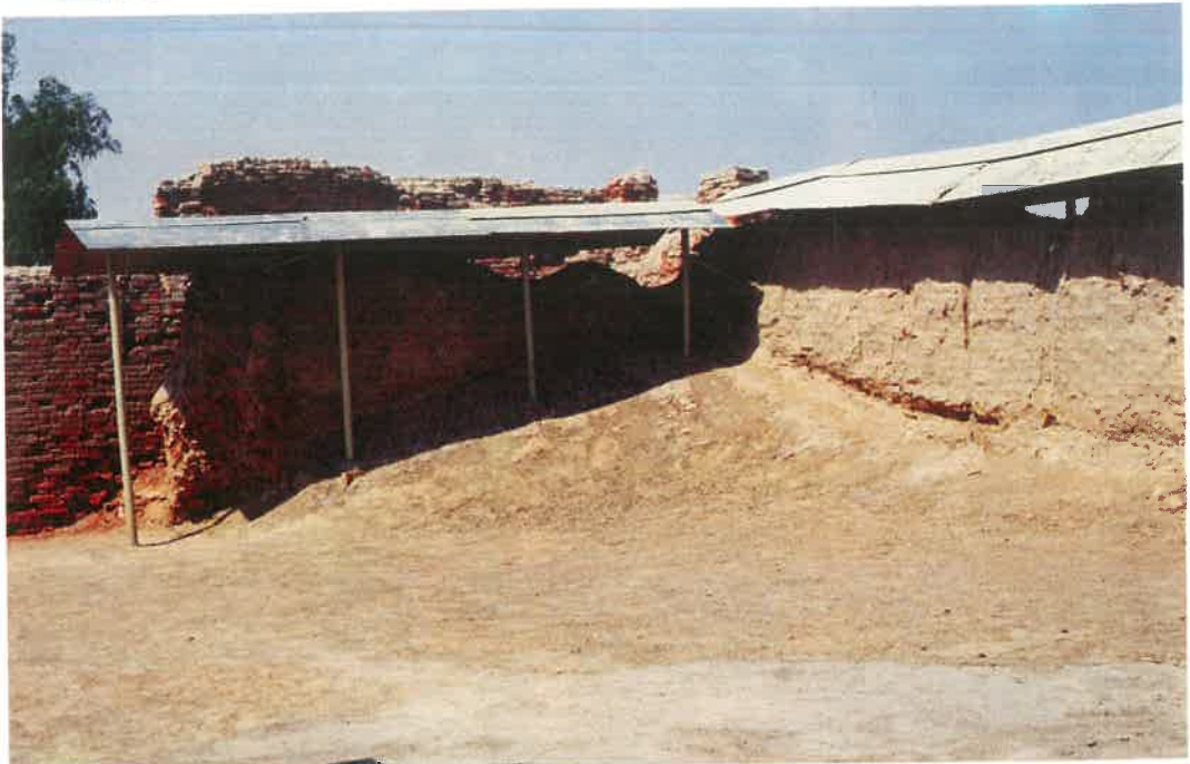
Mudbrick wall conserved by providing cover
