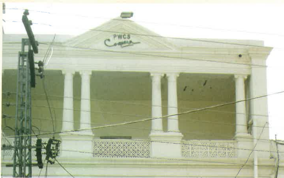
Fig. 136: Front view of first floor of Coopera Art Gallery-2016.
