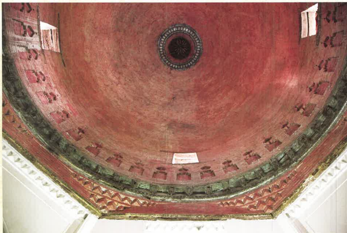
Interior view of dome.
