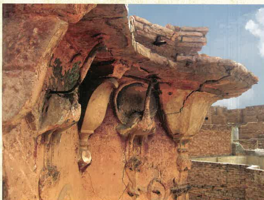
Detail of parapet.
