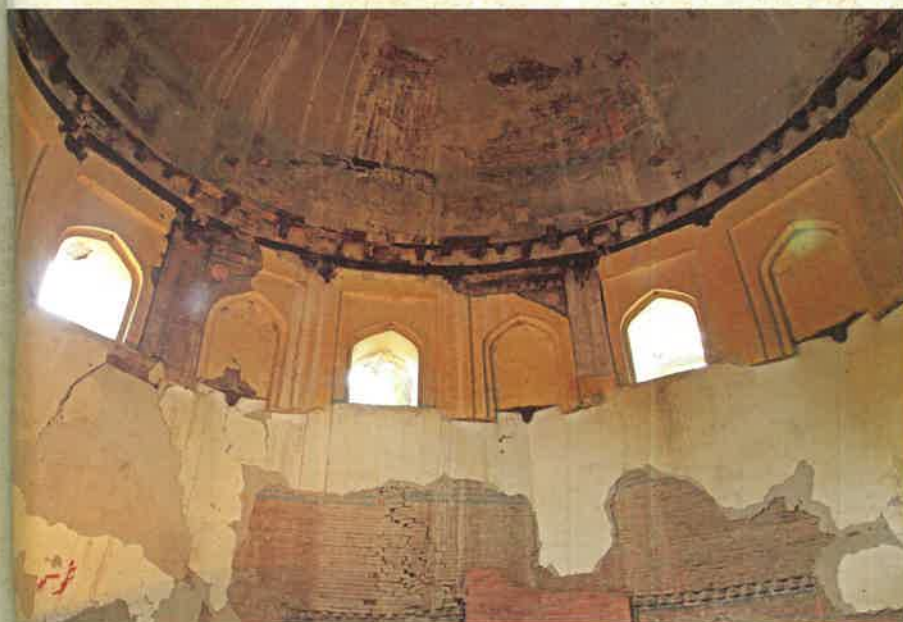
Interior view of dome.
