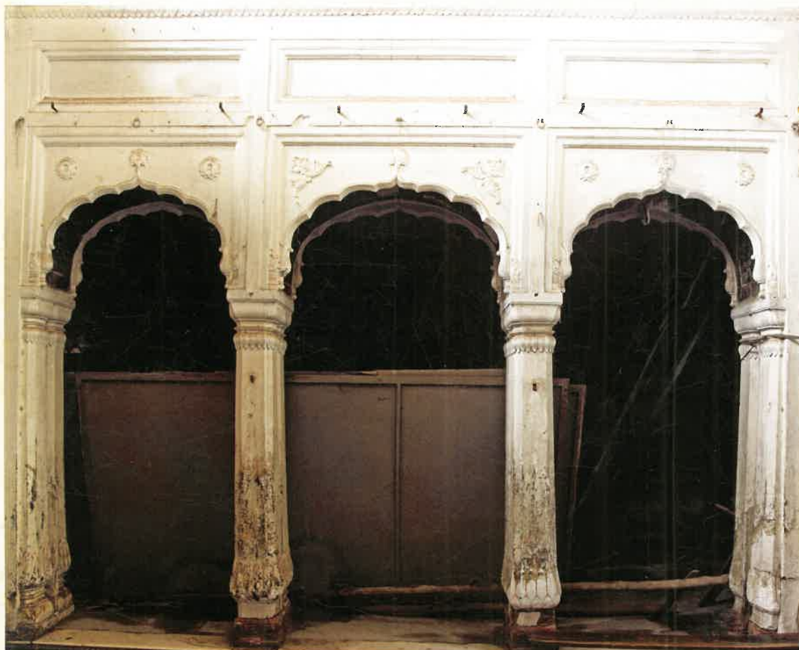
Verandah on the ground floor of Main Hall.
