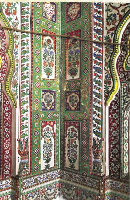
Corner detail of internal wall.
