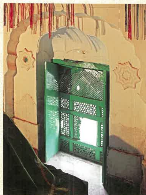
Wooden fret work in opening.
