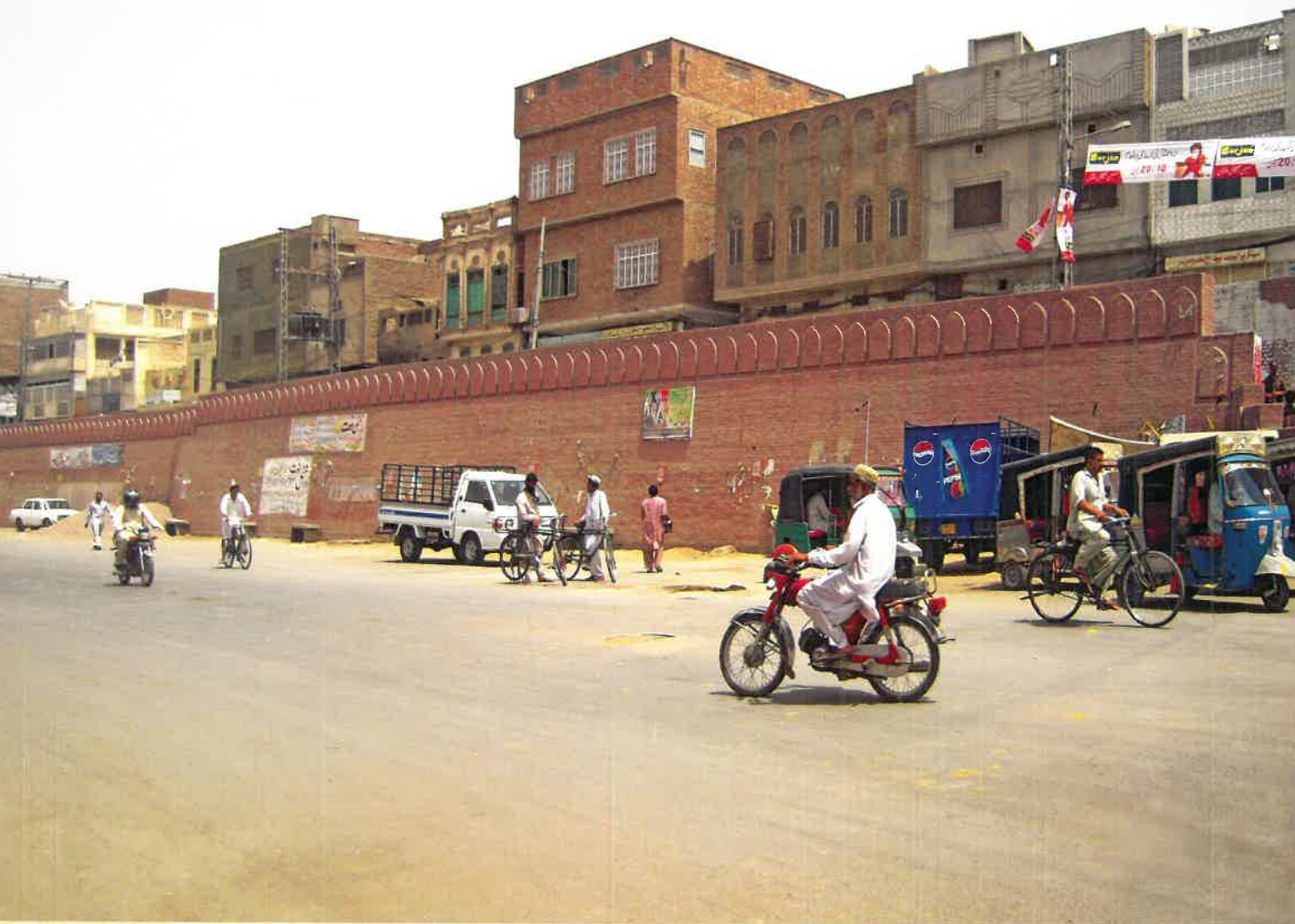
View of the reconstructed wall along the south Circular Road.
