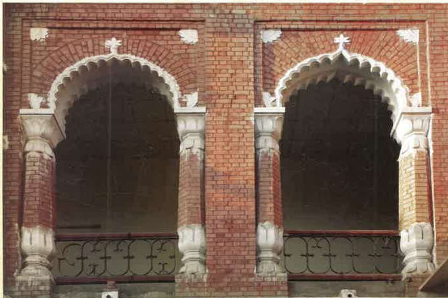
Detail of corridor arches.
