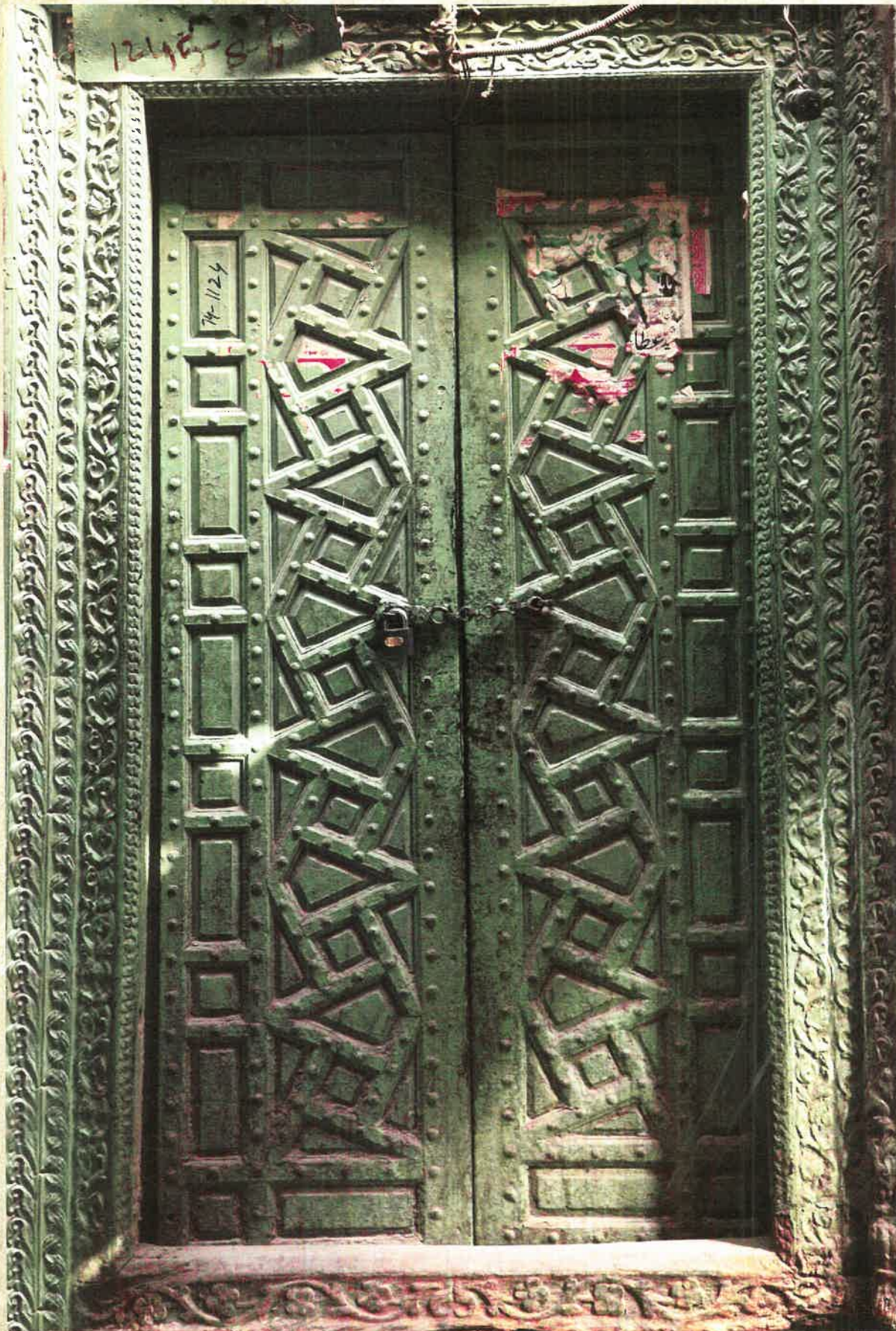
Door detail on the ground floor.
