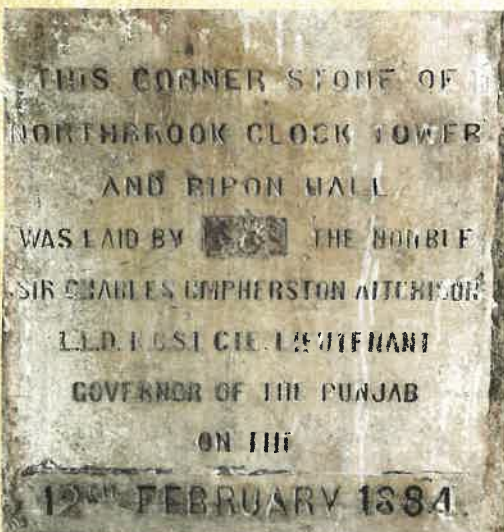
Inauguration plaque inside the entrance.
