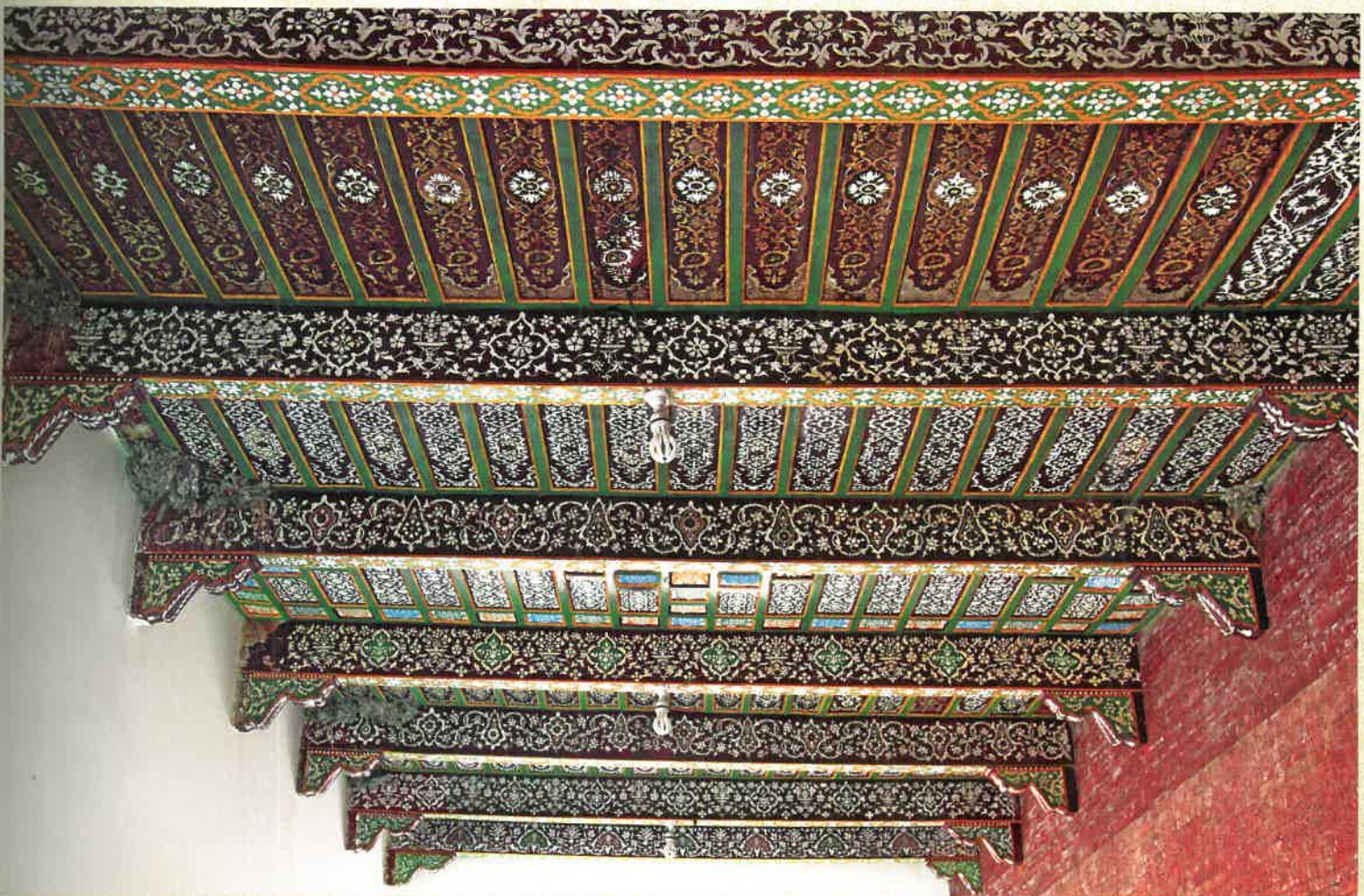
Roof Details of verandah.
