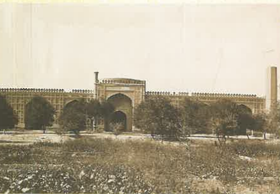
Photograph of Eid Gah with collapsed dome and minarets by William Henry Baker, 1865. (Courtesy: British Library)
