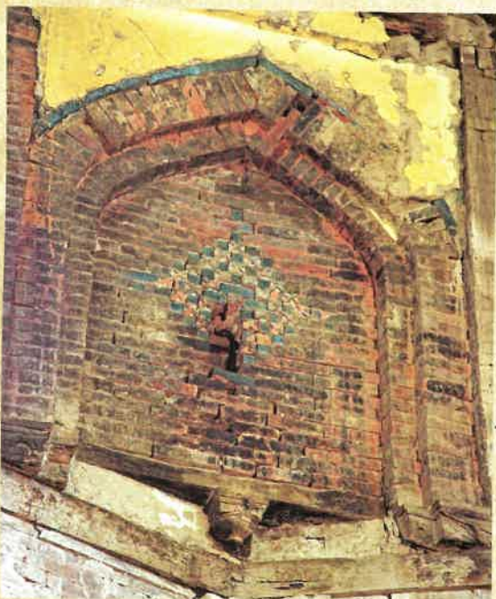
Tile and masonry detail.
