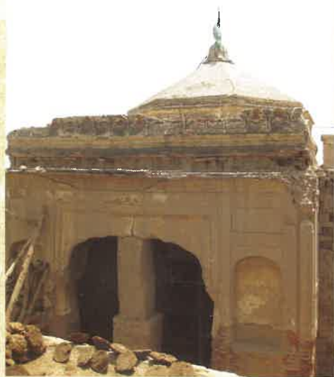
Condition of Mandir.
