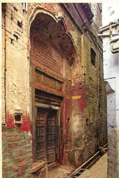
Main entrance from the street.
