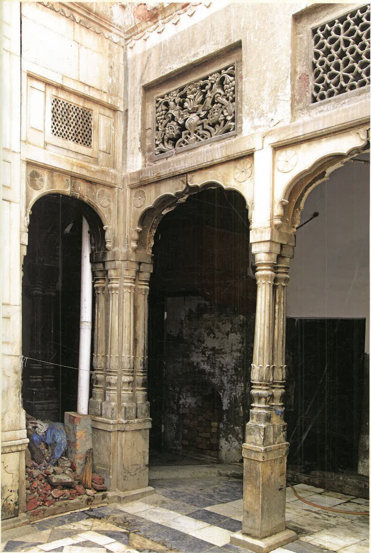
Veranda columns detail.
