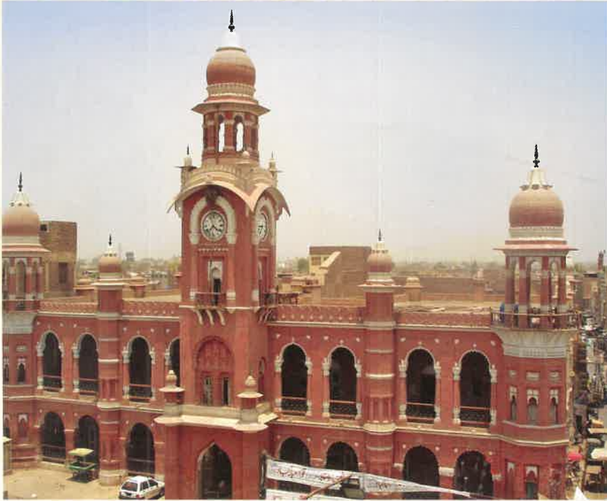
Main façade of Ghanta Ghar.
