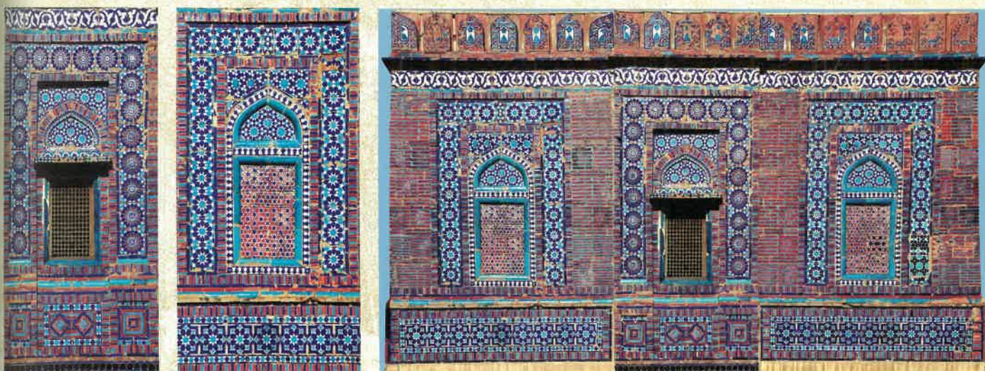
Detail of tile work.
