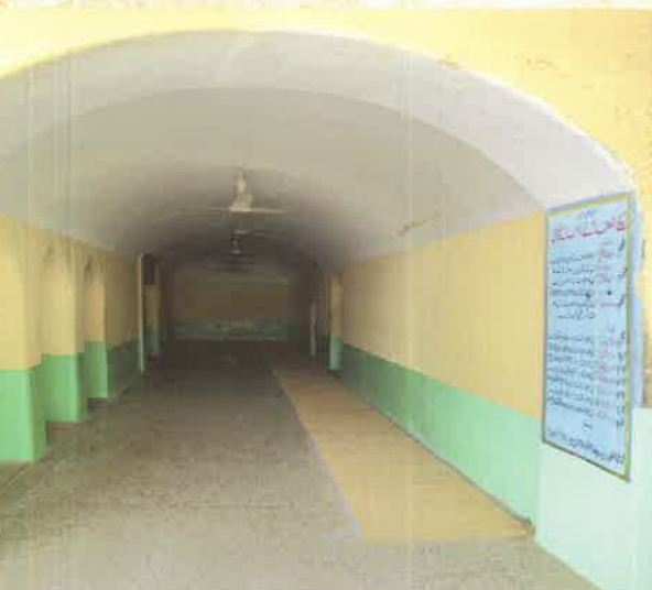
Vaulted verandah on the west of the Shrine.
