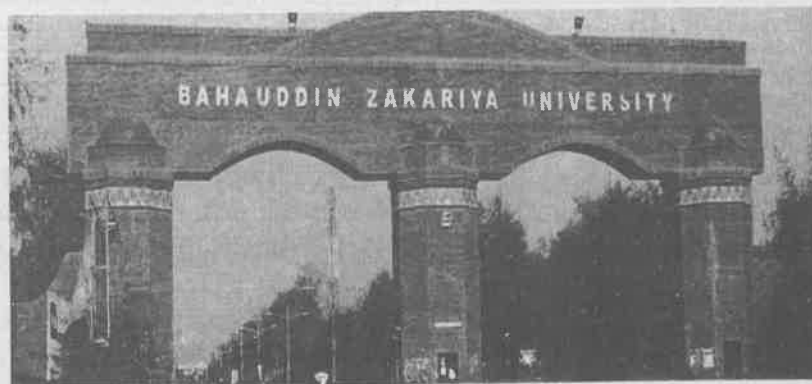
Fig. 120: Main Gate of the Bahauddin Zakariya University, Multan.
