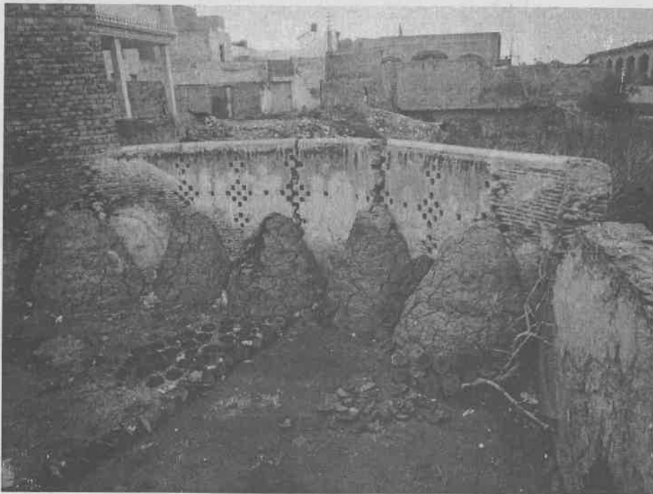
Fig. 78: Suraj Kund crude buttresses have been created to support the walls..
