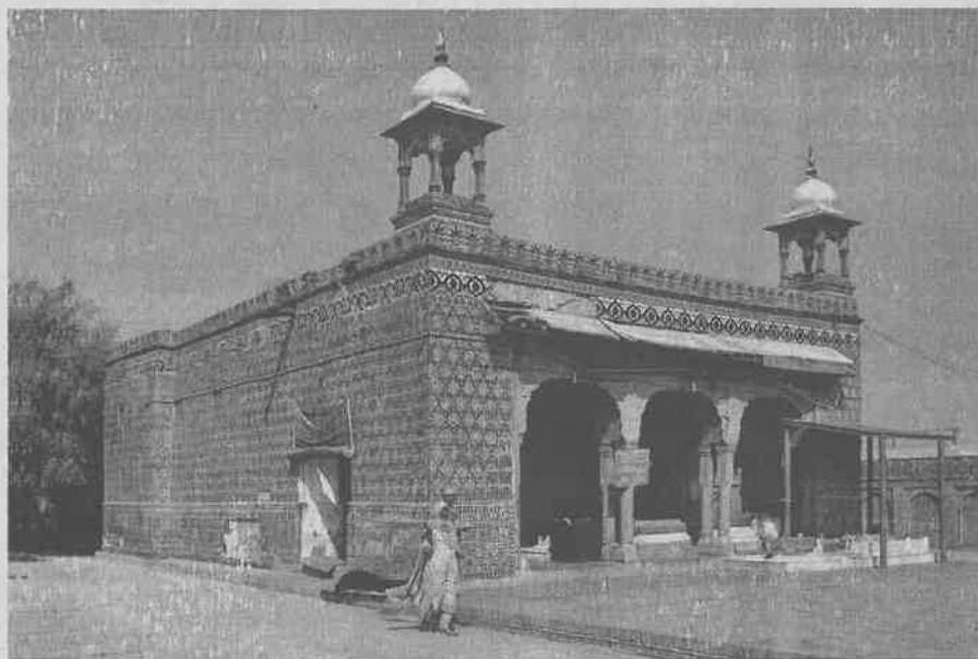
Fig. 172: Tomb of Bibi Pak Daman is rectangular in plan building without any dome. It has a kiosk at each corner on the front. The entrance is made of a veranda with three multi-cusped arches all made of wood and painted green.
