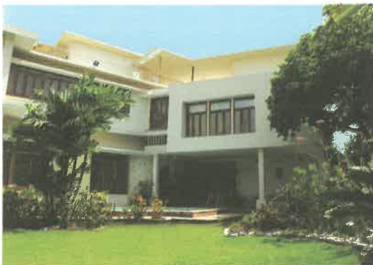
Jamil House with garden, Karachi, 1959-60 (First floor subsequently added by owner)
