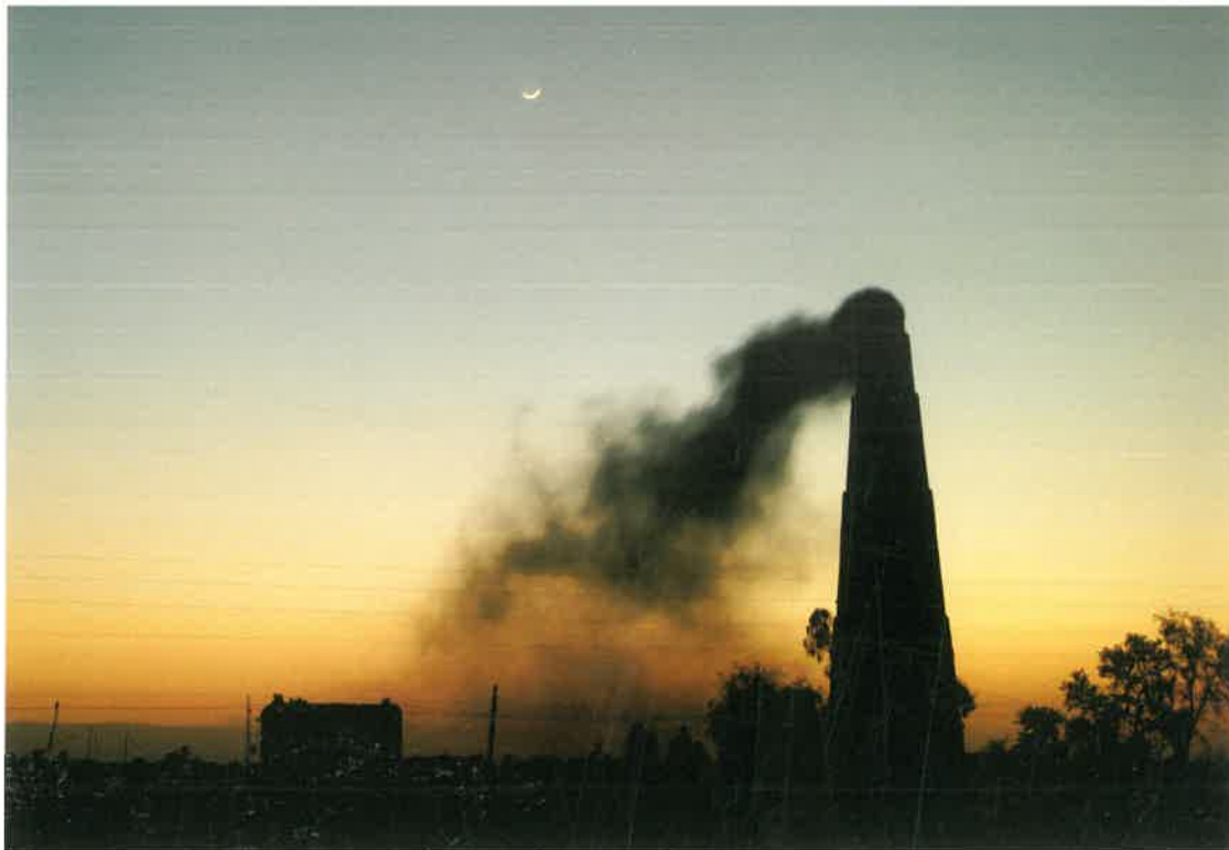
Brick-kiln emitting smoke, indicating development in progress in Haripur area.
