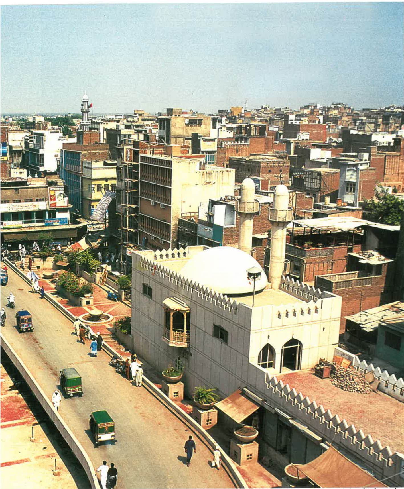
An aerial view of Peshawar city.
