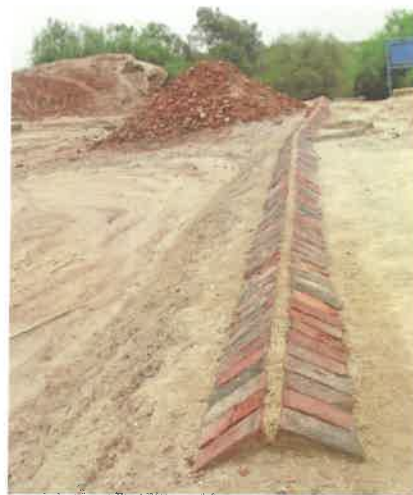
Harappa: Covered Drain.
