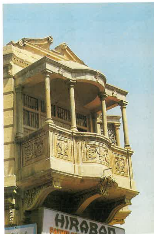
Stone built balconies projected over corinthian style brackets, Hyderabad.
