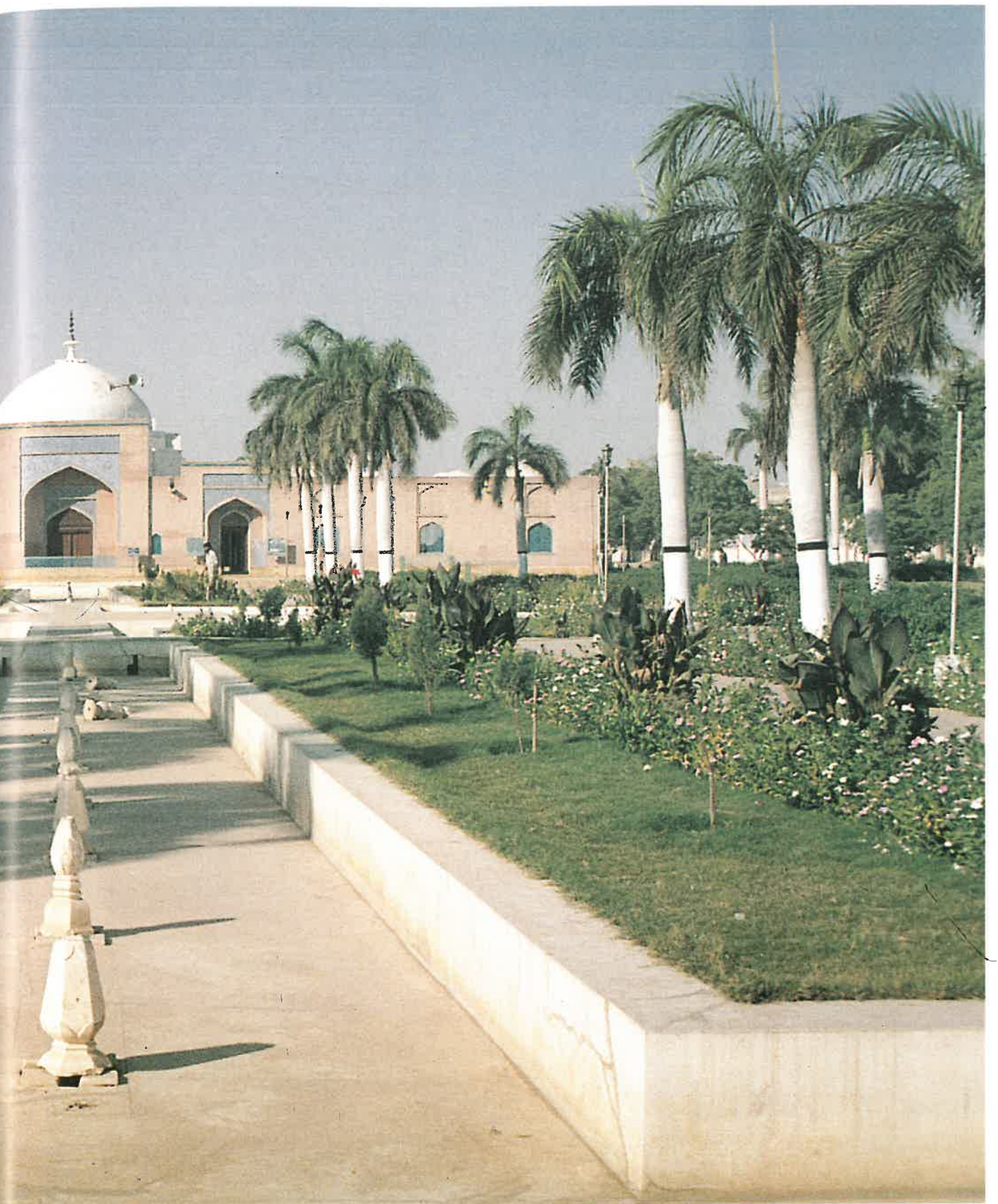
Shahjahani Mosque, Thatta -- General View.
