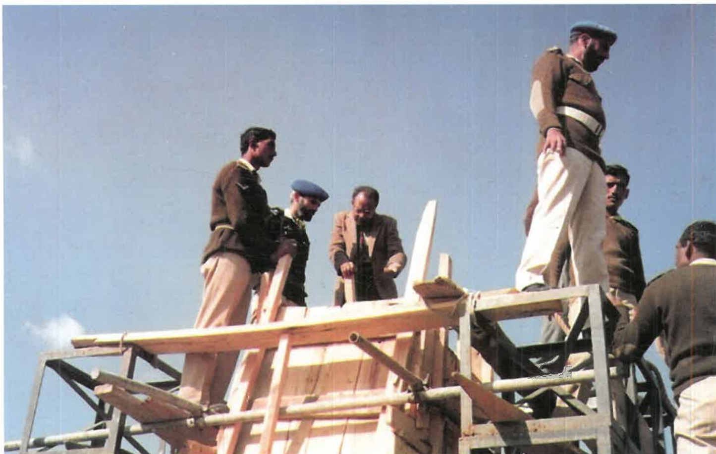
Rahi directing Pakish Military Personnel during the installation of the Faith First Monument PMA - Kakul, 2005
