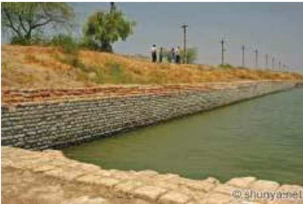
Figure III.1.29 Lothal Dockyard. ( http://www.shunya.net/Pictures/WesternIndia/Gujarat/Lothal/Lothal.htm ).
