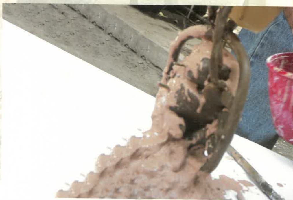
Fig. 30 - Outer cover with plaster 2 parts, brick dust 1 part and grog 1 part
