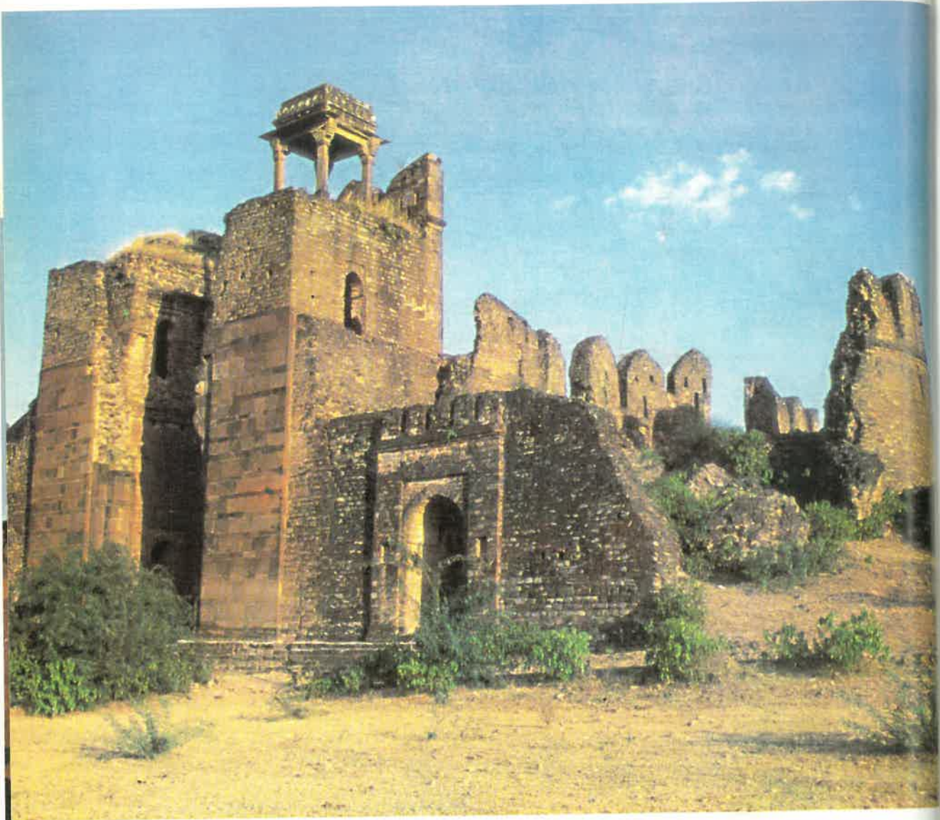
Shah Chandwali Gate.
