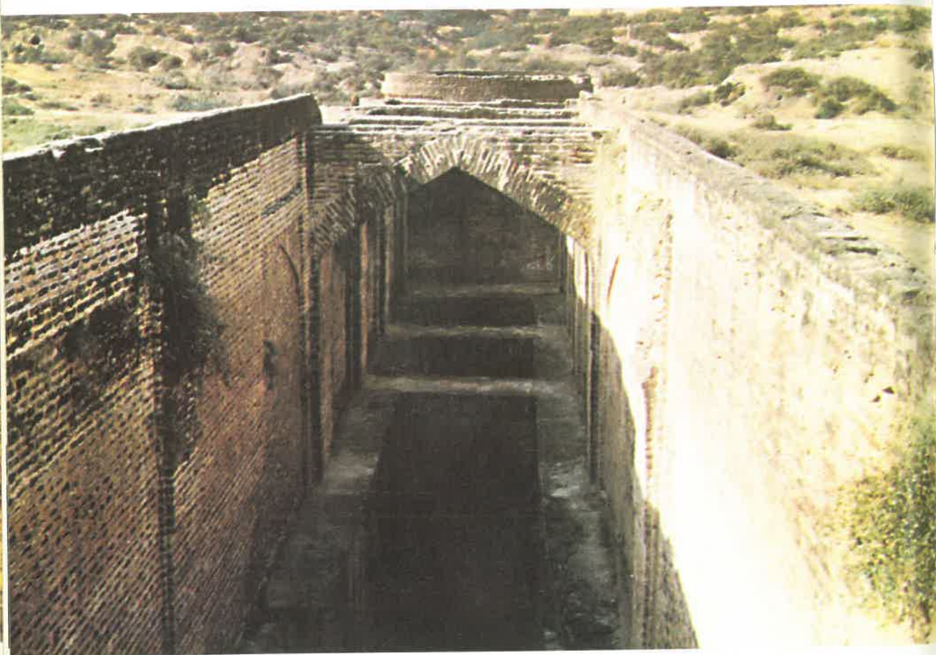
Interior view of Baoli near Tulla Mori Gate.
