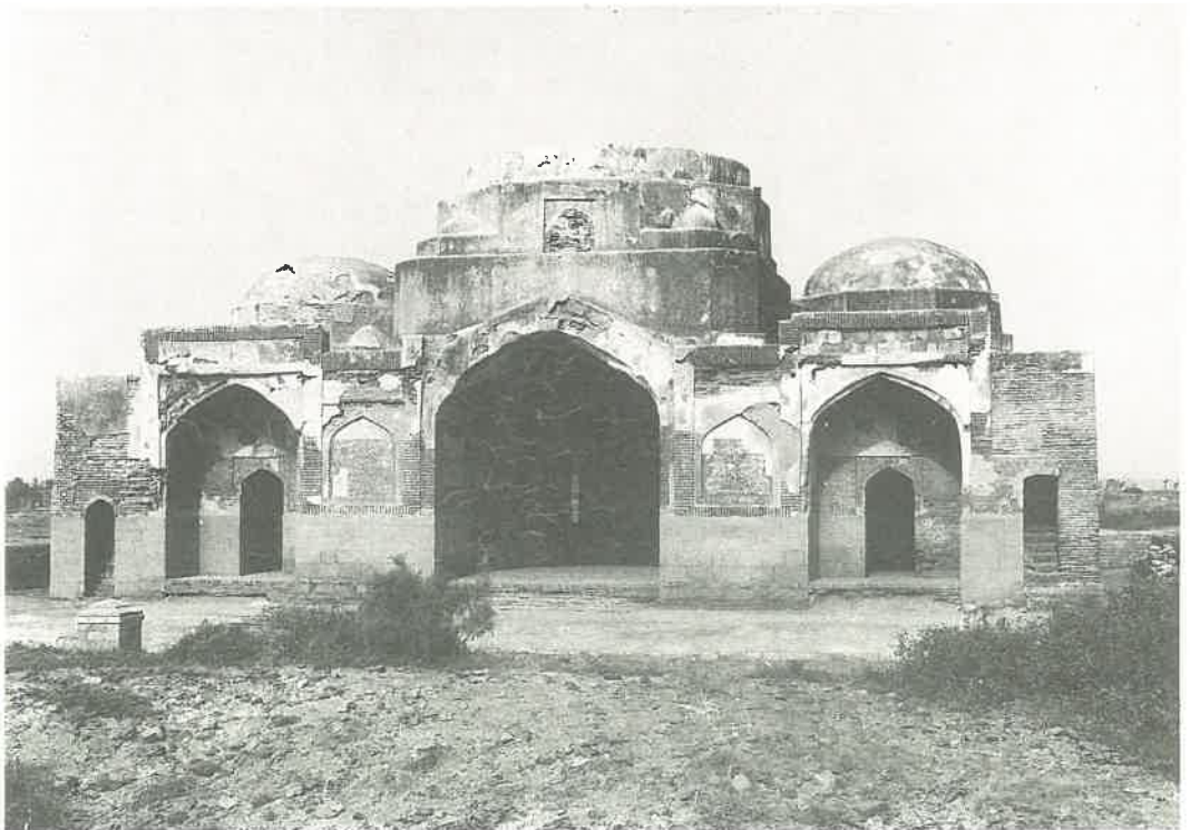
Pl. 34 : Thatta: Dabgaran Mosque - General view.
