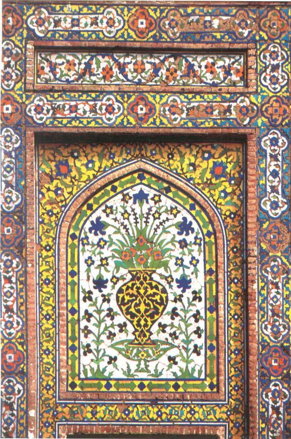
Fig. 380 Panel on gateway. Rectangular panel with blind recessed arch, cut tile mosaic depicting floral blooms.
