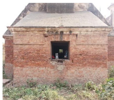
Figure 5-19: Image showing structural damages such as peeling of lime plaster and rotten bricks
