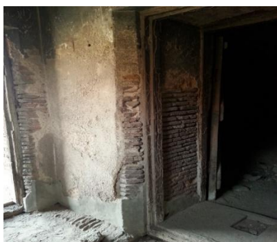
Figure 5-19: Image showing structural damages such as peeling of lime plaster and rotten bricks
