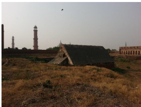
Figure 5-18: Image showing the context of Barood Khana full of debris before conservation
