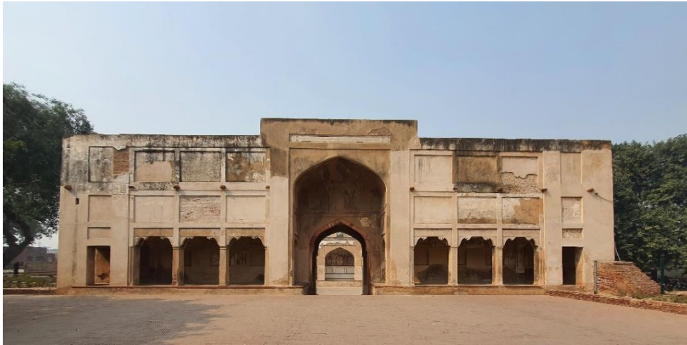
Figure 33: Eastern Entrance View of Makātīb Khāna, Lahore Fort.
