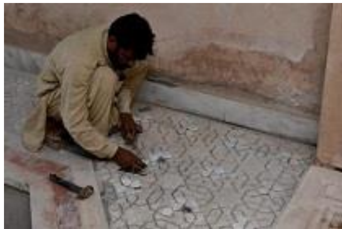
Figure 157: An Artisan is fixing the Floor Tessellation marble. Source: Archeology Department of Punjab.
