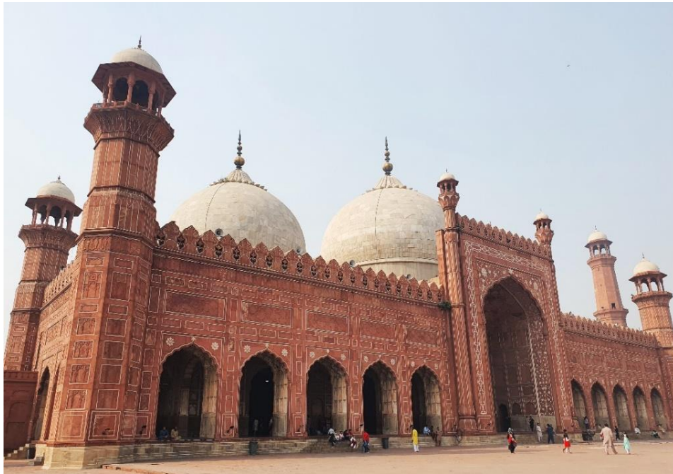
Figure 170: Facade of Bādshāhī Mosque Lahore.
