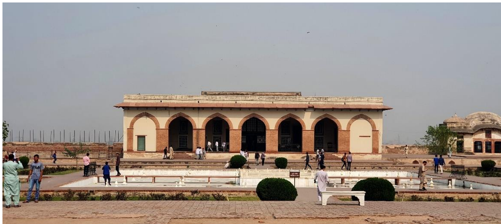
Figure 42: View of Bari Khawābgāh in Jahāngīr's Quadrangle.
