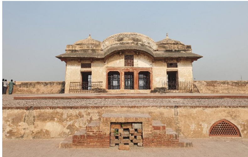
Figure 43: Sih-dari inside Jahāngīr's Quadrangle, Lahore Fort.
