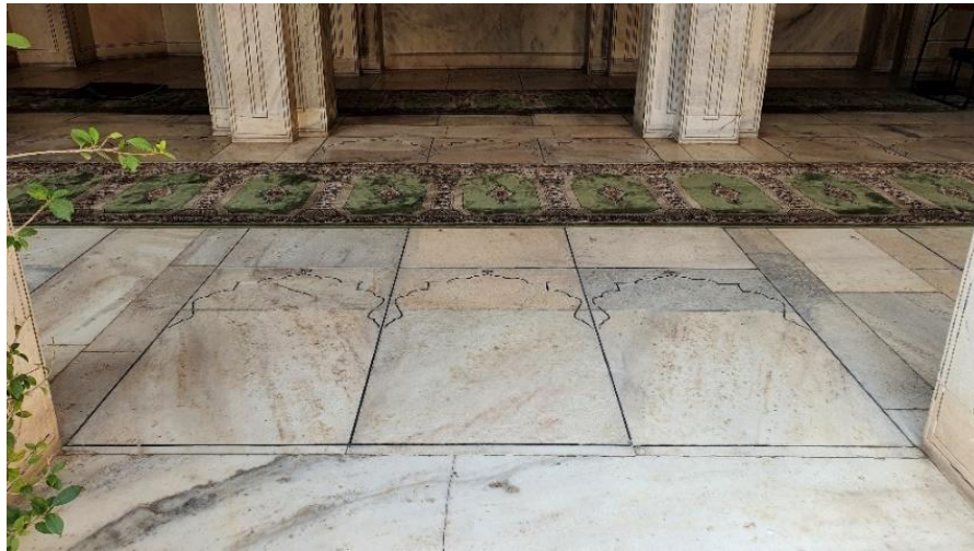
Figure 32: Black Stone Lining for Muṣallā on the Floor of Motī Masjid.
