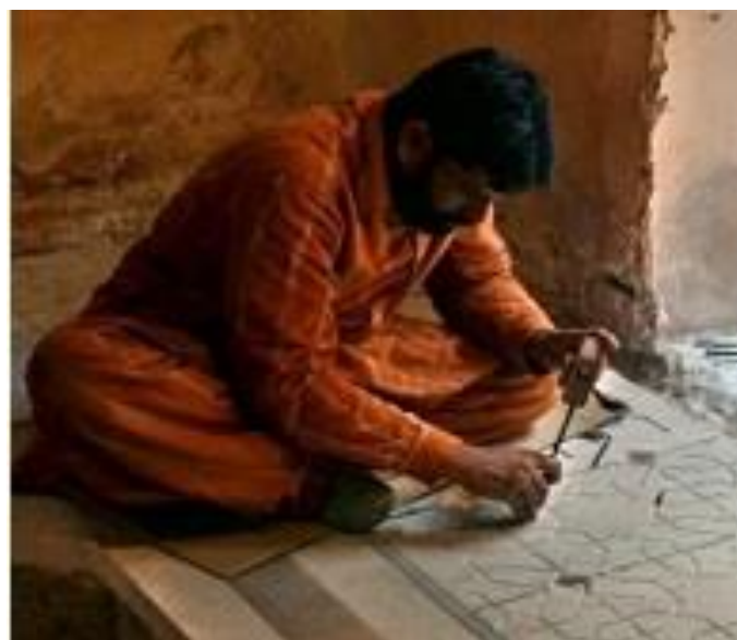
Figure 158: An Artisan using the Traditional Chisel and a Hammer on the Surface of Tessellated Floor. Source: Archeology Department of Punjab.
