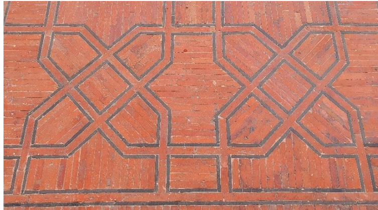
Figure 148: Brick floor of Wazir Khan Mosque Lahore.
