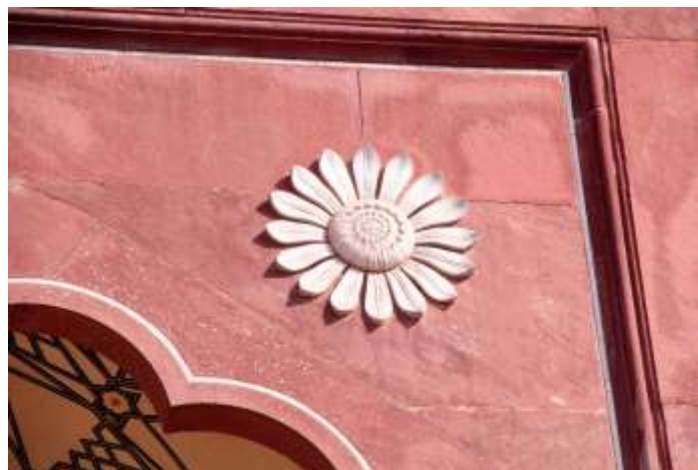
Fig. 34. Sunflower of white marble inlaid in red stone on the spandrel at the backside of main entrance arch.
