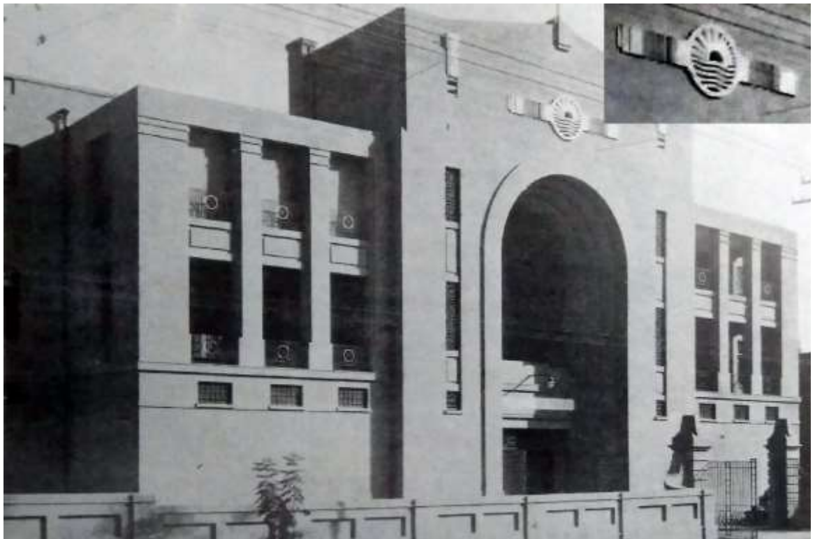
Figure 3.61. The Façade of the Complete Police Station photograph, 1937, Lahore Recollected an Album by F.S. Aijazuddin, p 178.
