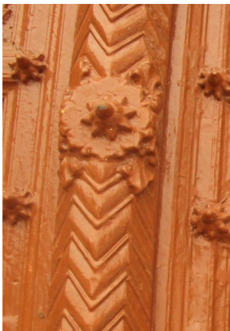
Plate 183 Close up of the central bar of the door of Gurudwara Dera Sahib, Lahore (Photo by author)
